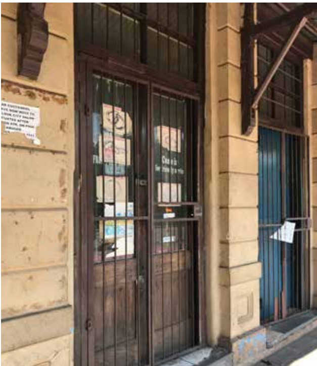
Fig 68. Closeup of timber door and facade details (Author, 2022)
