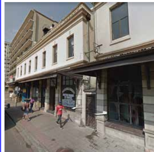
Fig 60. Trees removed and pavement cut short (Google Street View, 2019)
