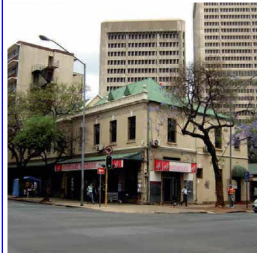
Fig 59. Before the widening of Paul Kruger St (Ashworth, 2008)
