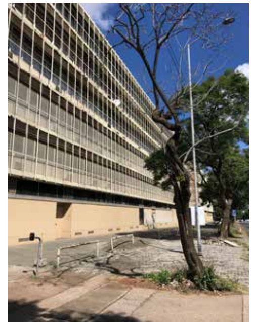
Fig 18. Struben St elevation of Department of Transport national administrative headquarters (Author, 2022)
