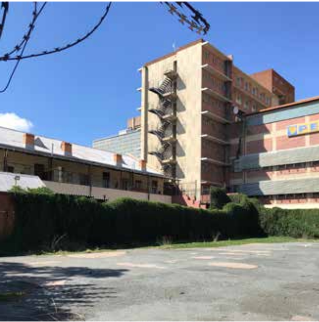
Fig 70. West elevation of Panagos Buildings (Author, 2022)
