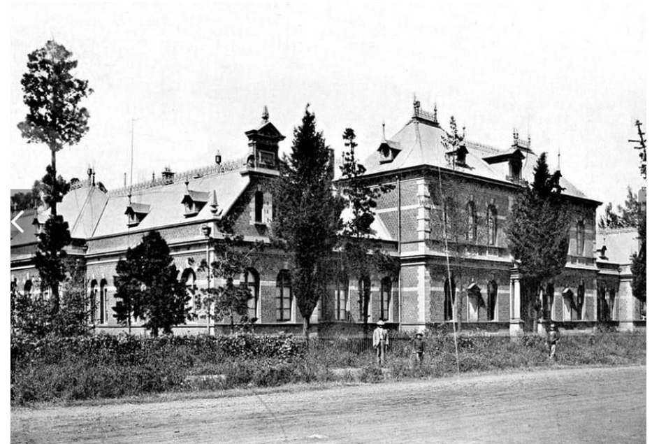
Figure 22 _ The demolished Staatsgymnasium ca. 1899 (Barker, 2014:138)
