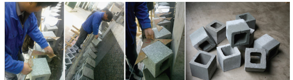
Figure 57 _ Teaching builders to use the templates (Yuan, Zhang & Han, 2013:146)
