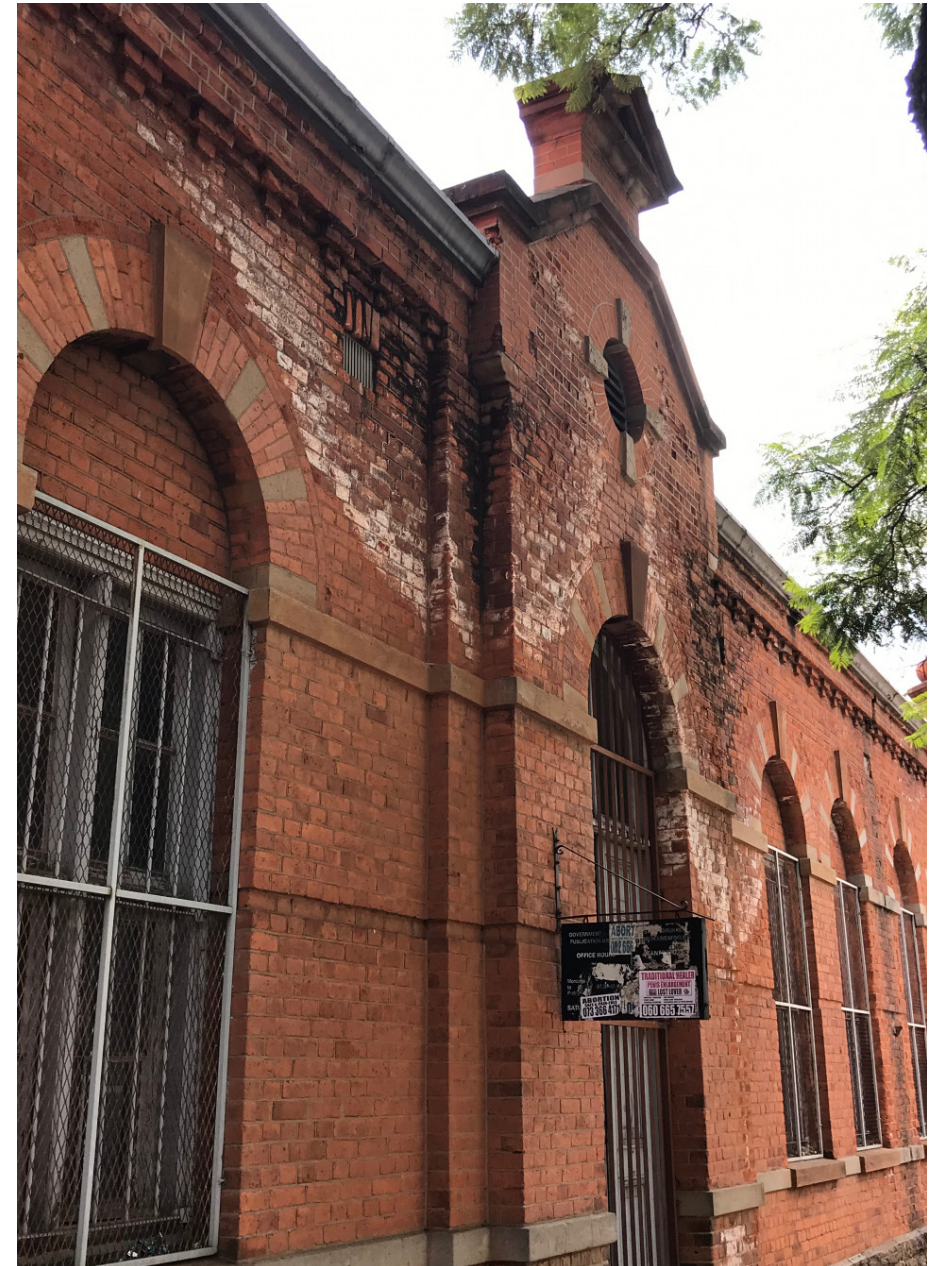
Figure 3 _ East facade of the Old Government Printing Works (Author, 2022)
