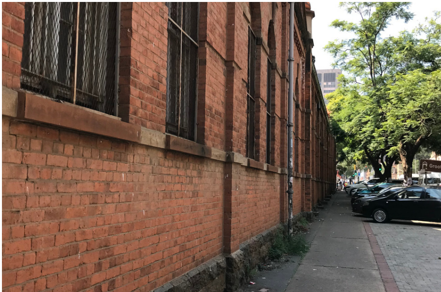
Figure 6 _ The barrier formed by the south facade (Author, 2022)
