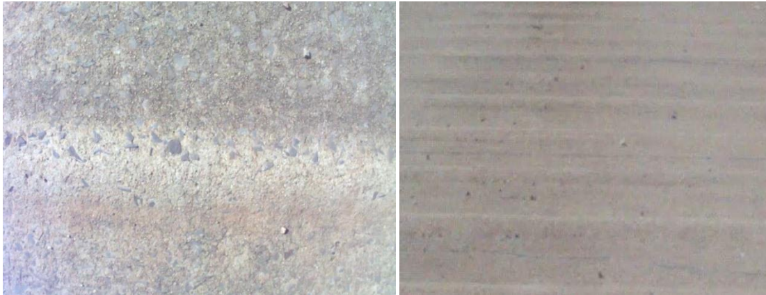
Figure 4.13: Straight corrugated road profile example of downward- and forward-facing data
