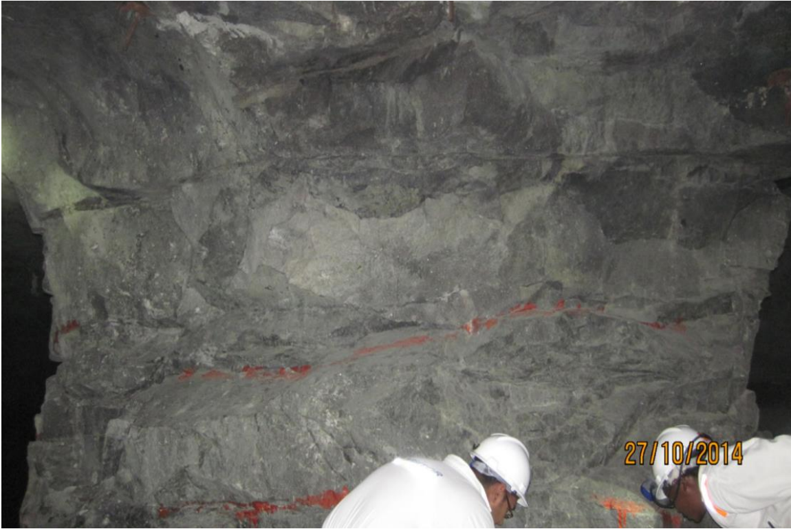
Figure 3-6. A pillar at Mine A showing the typical condition of the rock mass (courtesy N. Fernandes).
