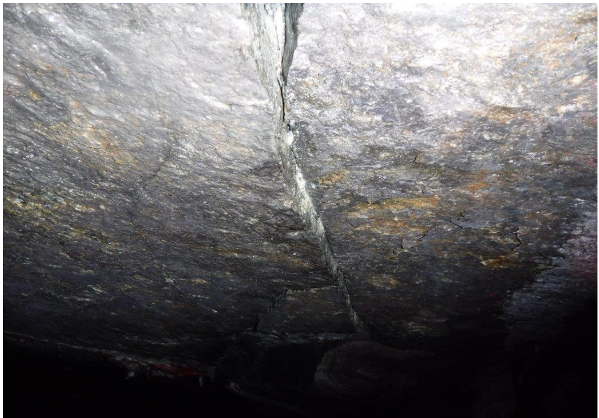
Figure 4-19. Tensile cracks in the hangingwall of the Level 5 failure zone.
