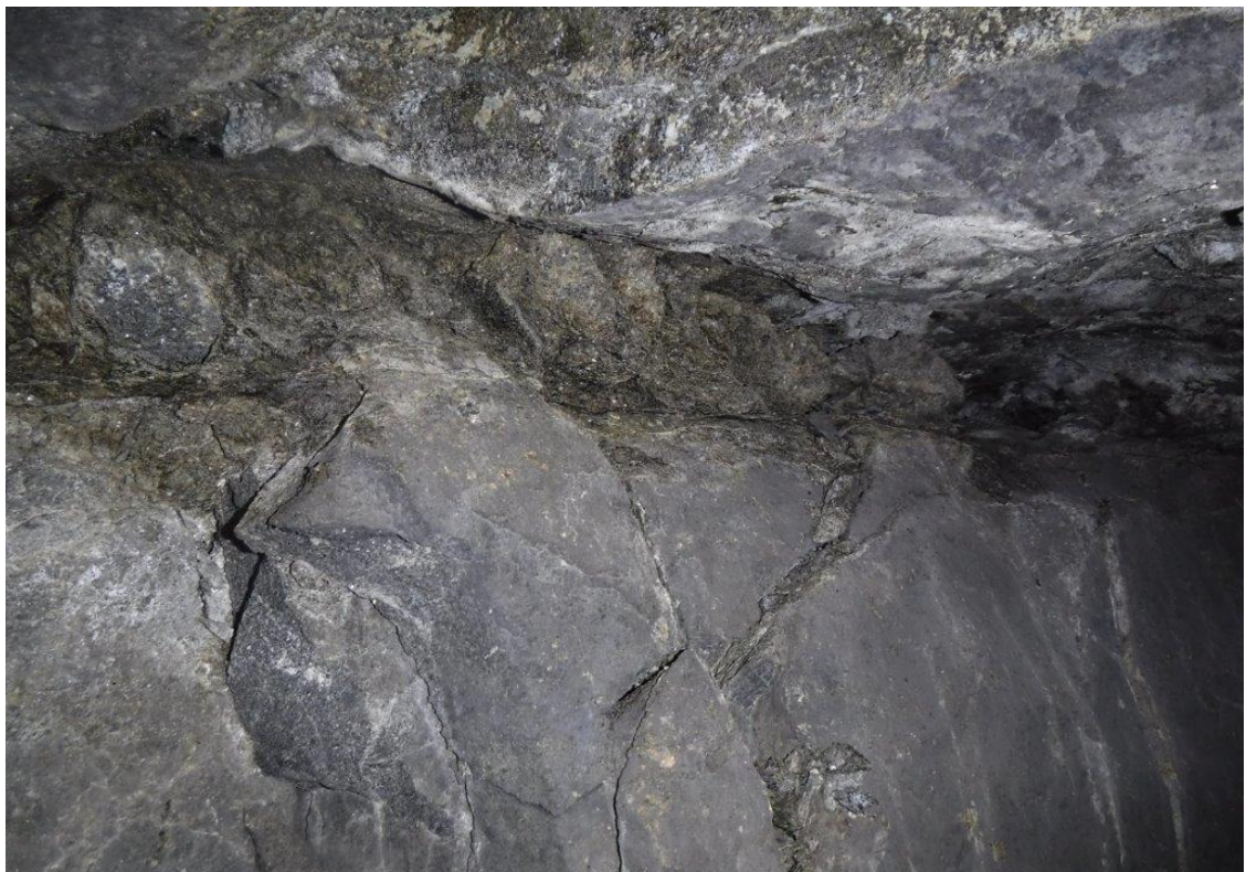
Figure 4-7. Position of the alteration zone in a pillar in the Level 3 failure zone. Note the thick alteration zone at the pillar/hangingwall contact.
