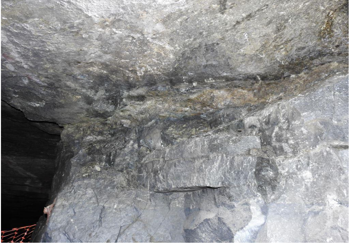
Figure 4-8. Another photograph of the nature of the alteration zone at the pillar/hangingwall contact.
