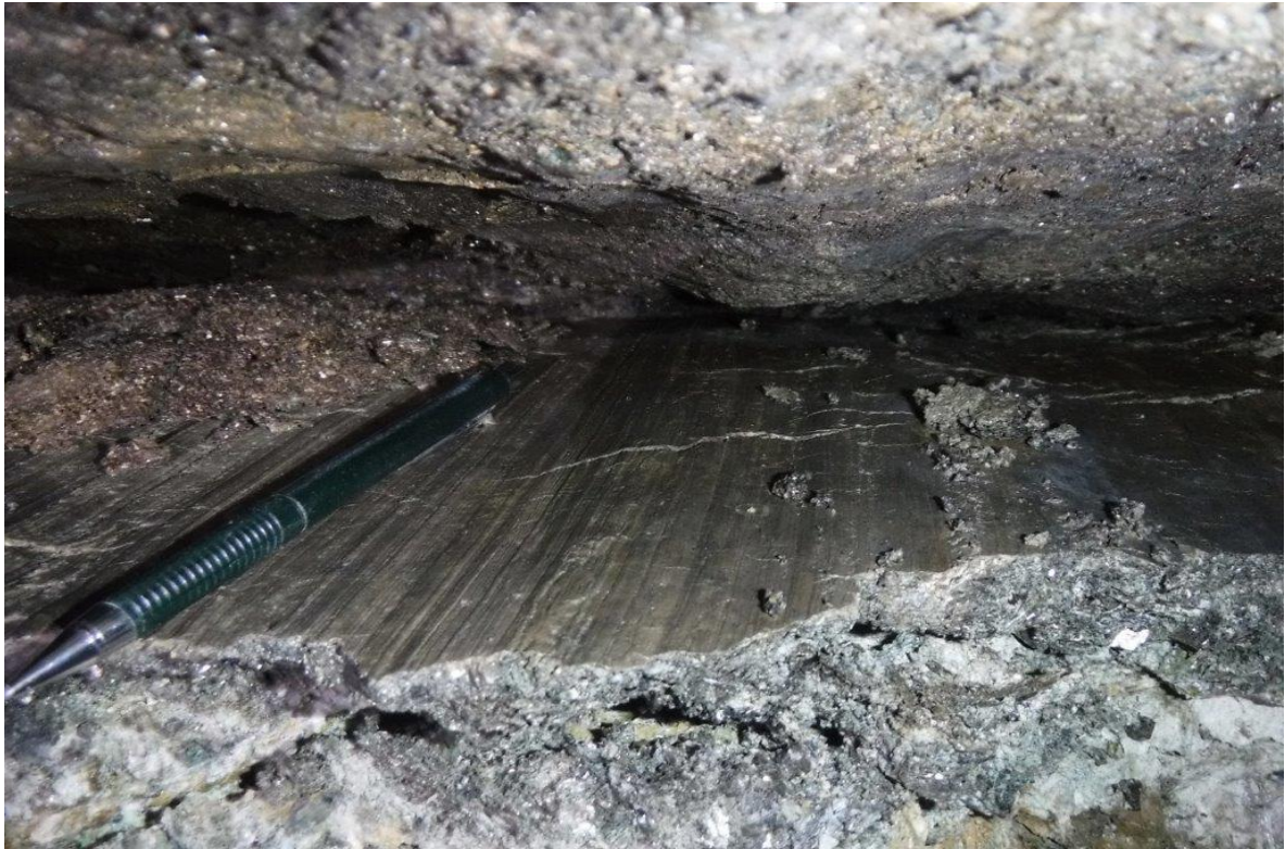
Figure 4-18. A slickenside surface between the crushed pillar material and the hangingwall.
