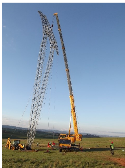
Figure 1 - Erection of a 400 kV type 520B guyed V-tower
