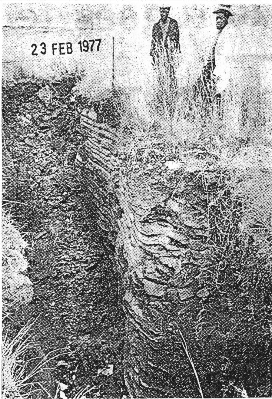
This sinkhole appeared close to a residential area in Laudium about three months ago. Despite complaints the council has taken no steps yet to fill the hole.
