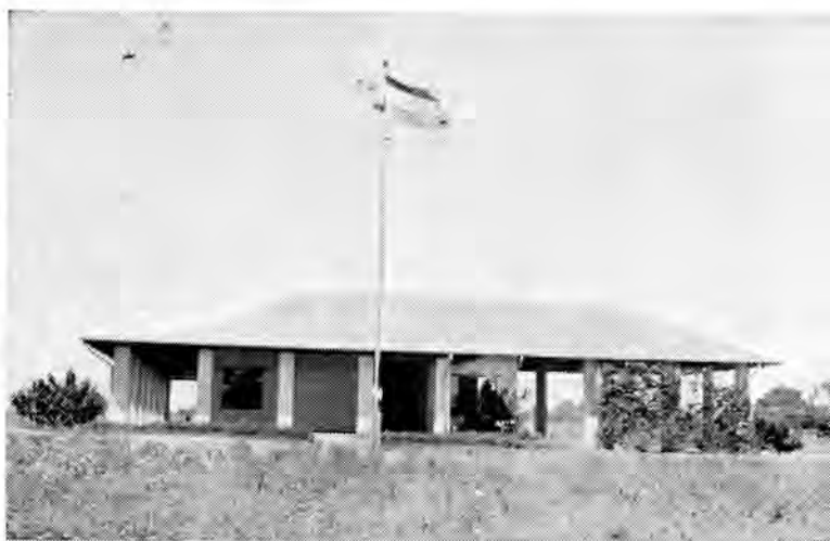
The Court House with the open Magistrate's Court on the right.
