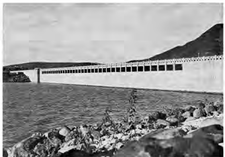
Van Ryneveld's Pass Dam near Graaff Reinet.
