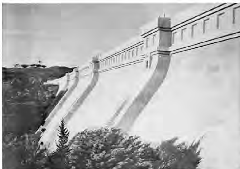
Kamanassie Dam, fifteen miles north-east of Oudtshoorn.
