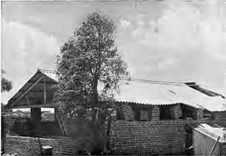
Photograph by Johansons Portrait Studio, Springs. Picture C. Partially rotated cowshed roof.
