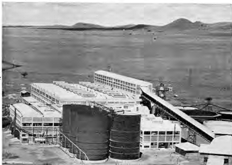
REDUCTION PLANT, LIBANON GOLD MINE
