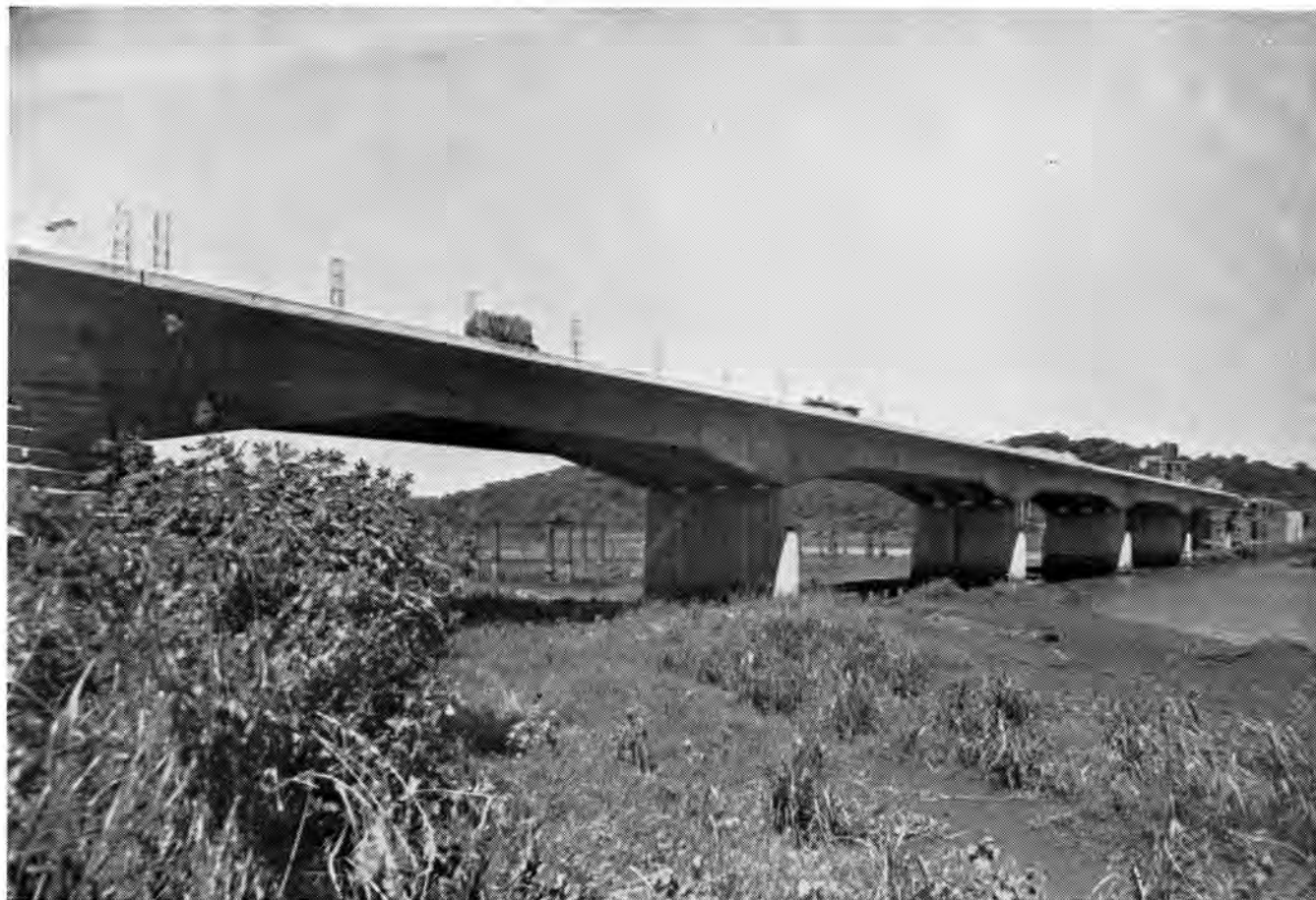
THE BRIDGE FROM THE LEFT BANK.
