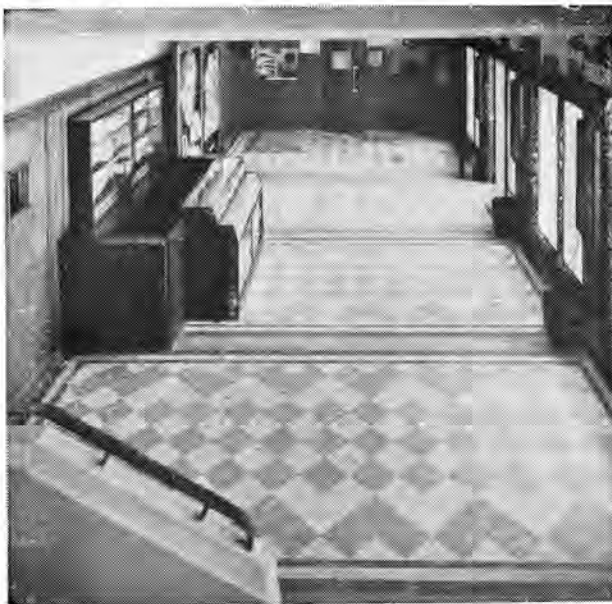
Entrance to Clarendon Cinema ... laid in Armstrong's Asphalt Tile ... by North British.
