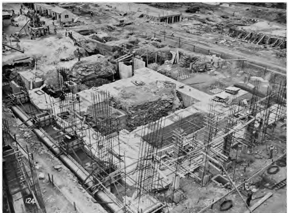
Looking north-east across the site of the new "B" station. The switch house foundations are in the foreground, with the new boiler house on the far side.
