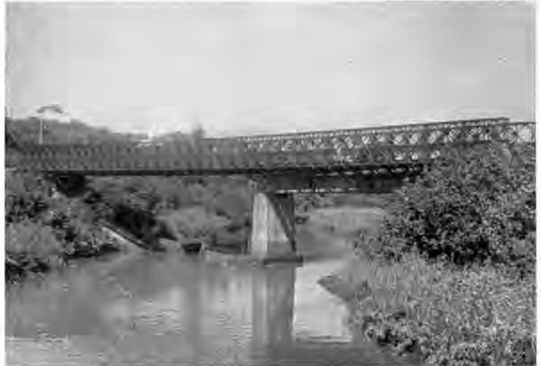
The temporary Bailey bridge, erected in ten days.
