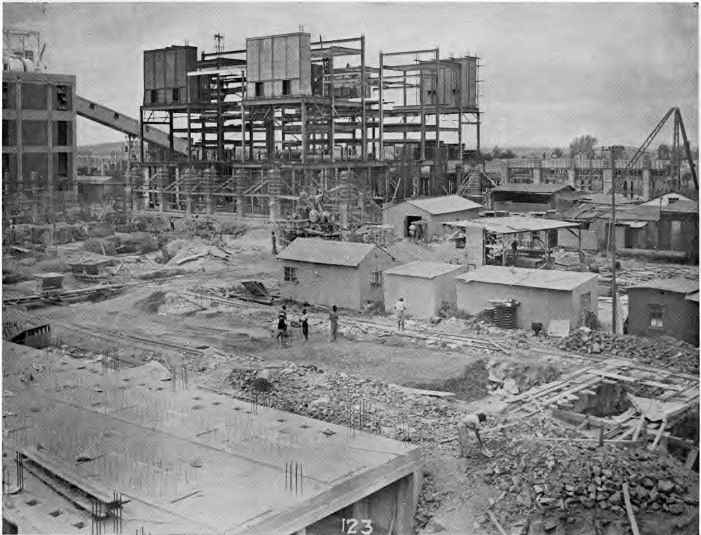
Looking north-east across the site of the new "B" station. The switch house foundations are in the foreground, with the new boiler house on the far side.
