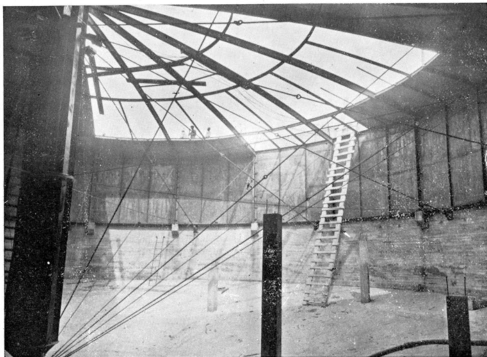
STEEL GASOMETER ROOF OVER SECONDARY DIGESTOR UNDER CONSTRUCTION.
