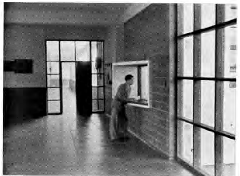
View of Public Entrance shewing enquiry counter set in a wall faced with 6 inch x 6 inch quarry tiles.
