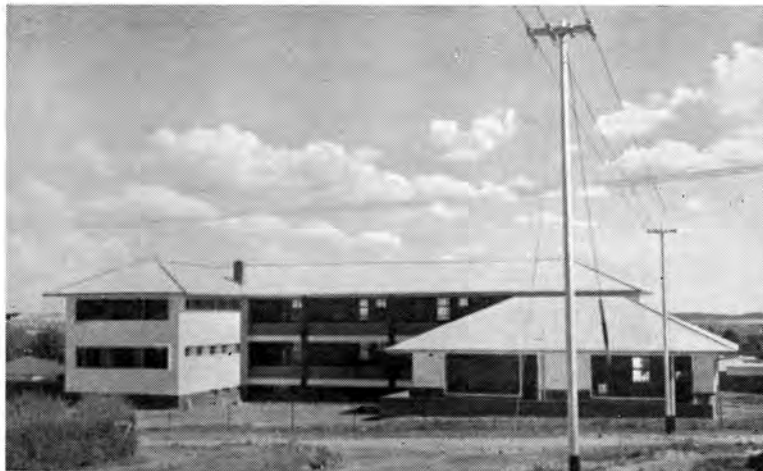
General View from the North.
