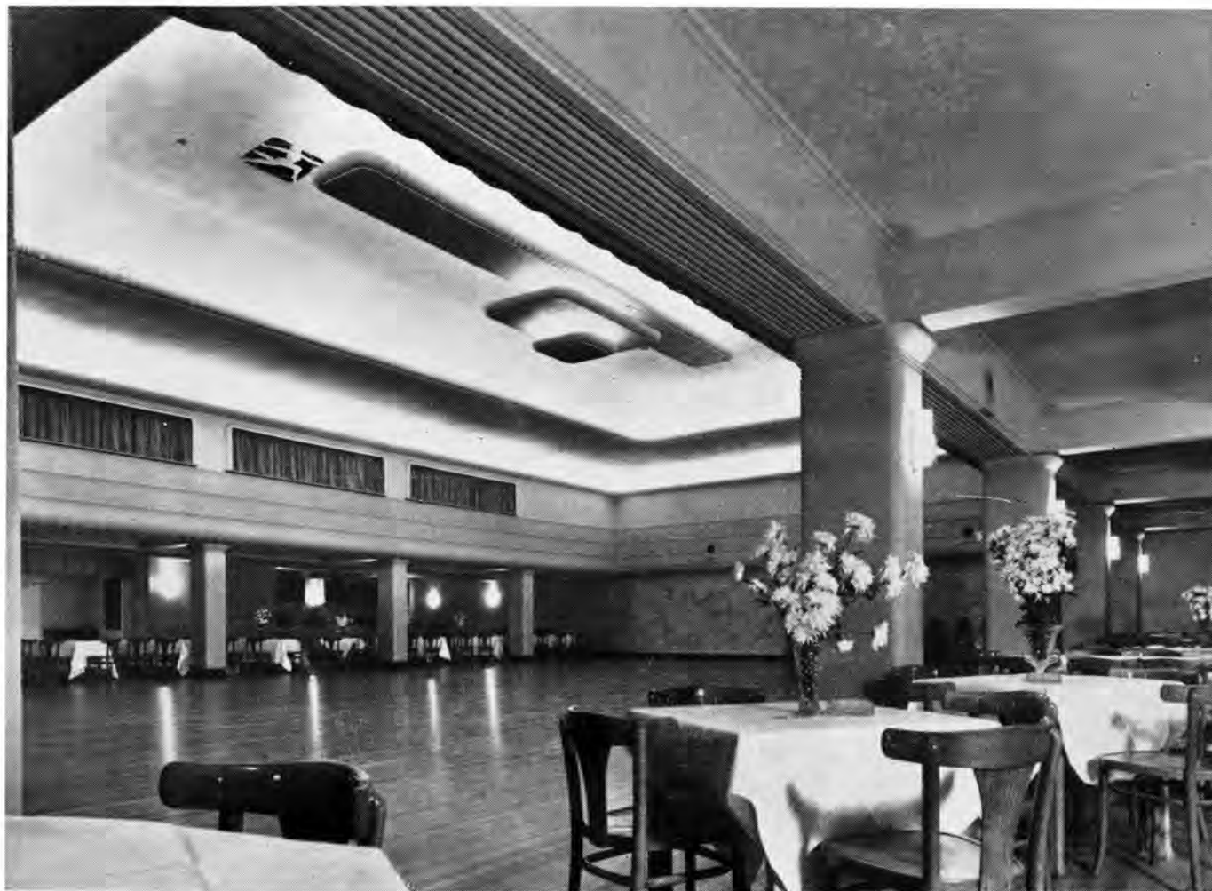
FIG. 6. A Ball Room illuminated by Cold Cathode Fluorescent Tubes.
