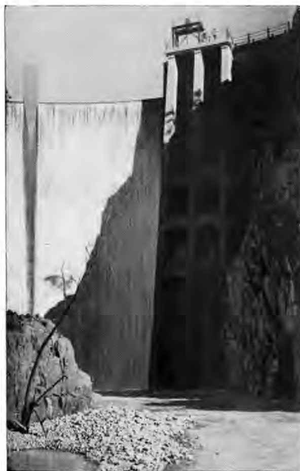
NJELELE DAM OVERFLOWING SHORTLY AFTER COMPLETION.
