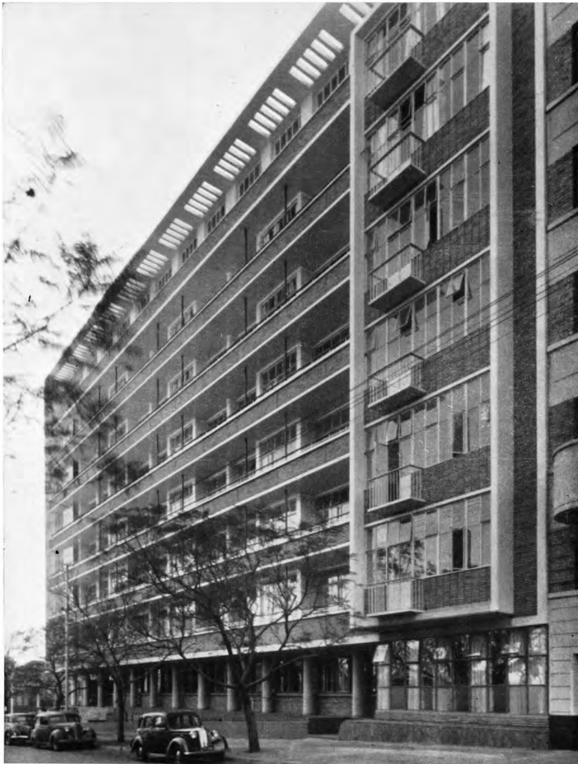
MAIN ELEVATION — TO ESSELEN STREET, JOHANNESBURG.
