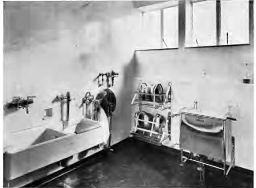
TYPICAL ARRANGEMENT ADOPTED FOR SLUICE ROOM.
