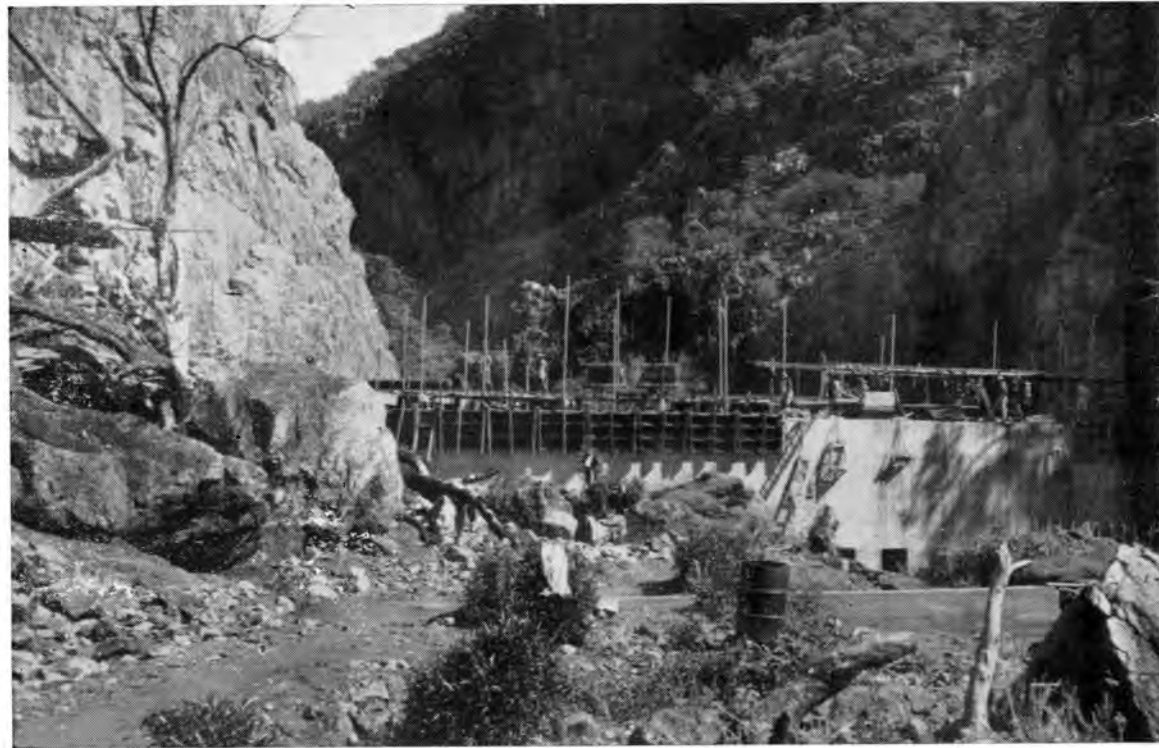
VIEW OF THE UPSTREAM FACE OF THE ARCHED WALL.
