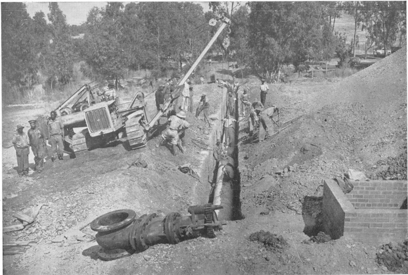
THE LAST LENGTH OF PIPE.
