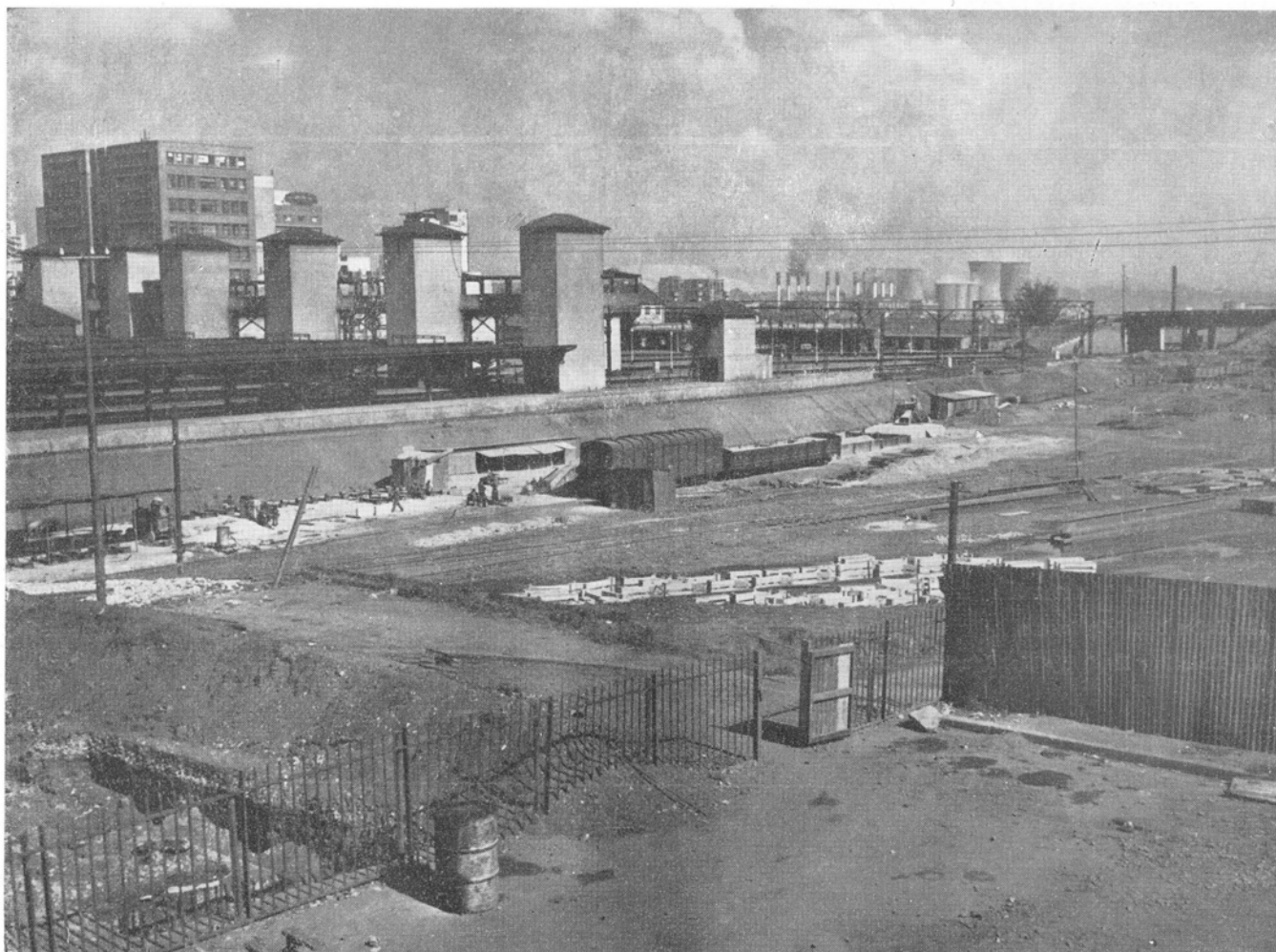
ACROSS THE EXCAVATIONS TO THE OLD STATION.
