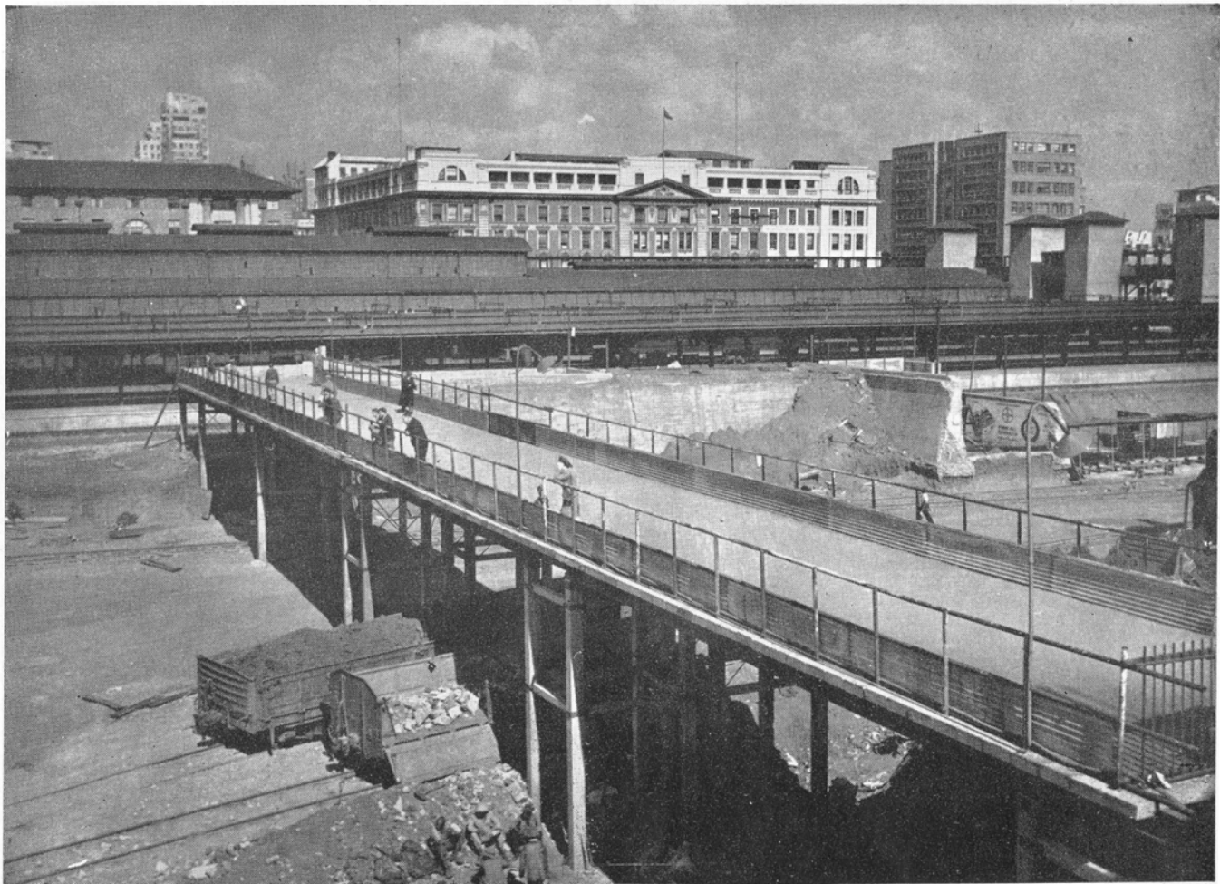
THE TEMPORARY FOOTBRIDGE.
