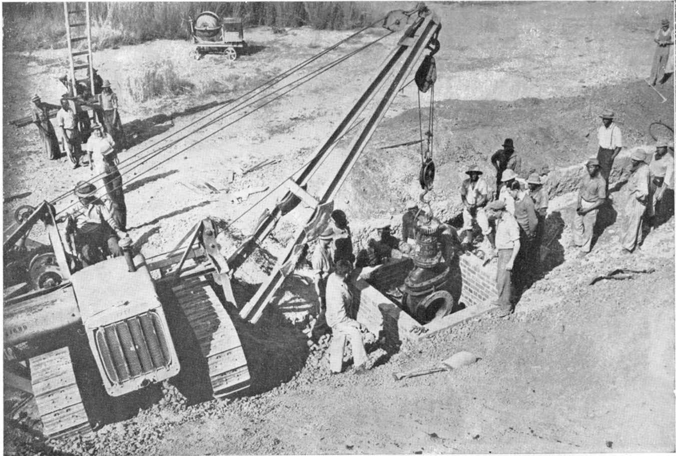
INSTALLING A VALVE.
