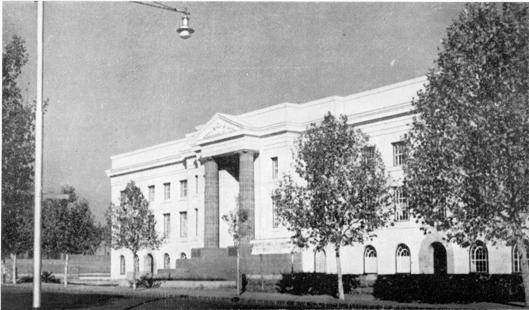
VIEW FROM THE NORTHWEST
