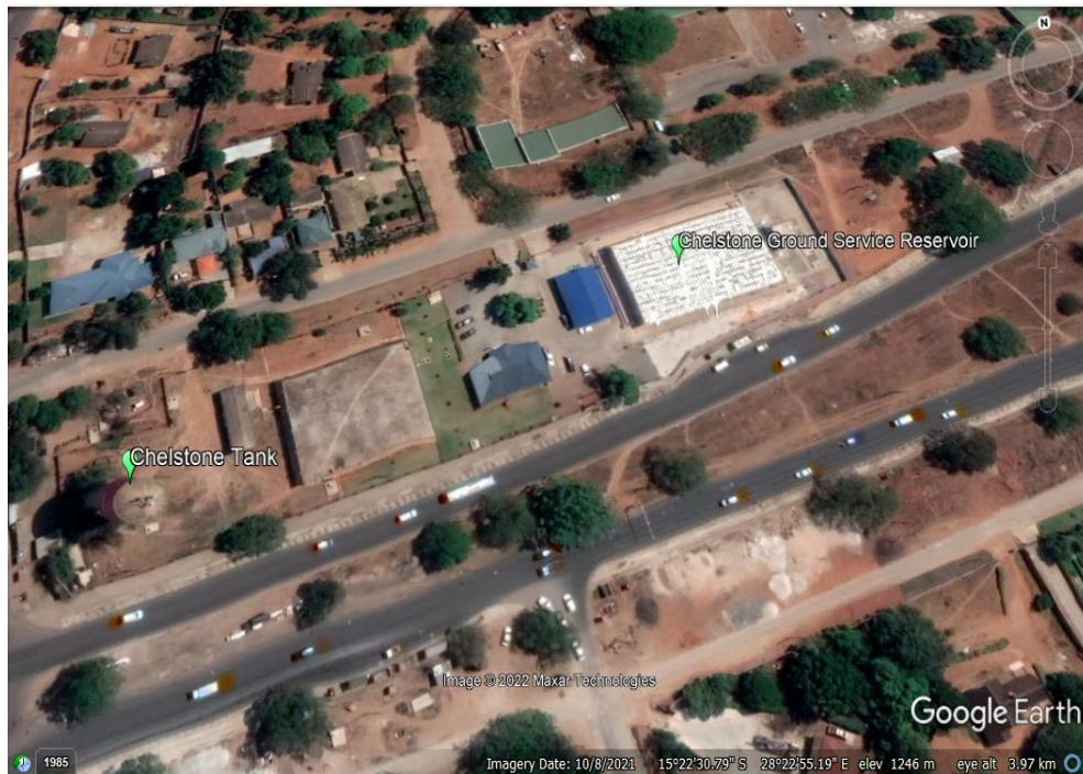
Figure 6-7: Location of the Chelstone Service Reservoir Site (Source: Google Earth Pro, 2022)
