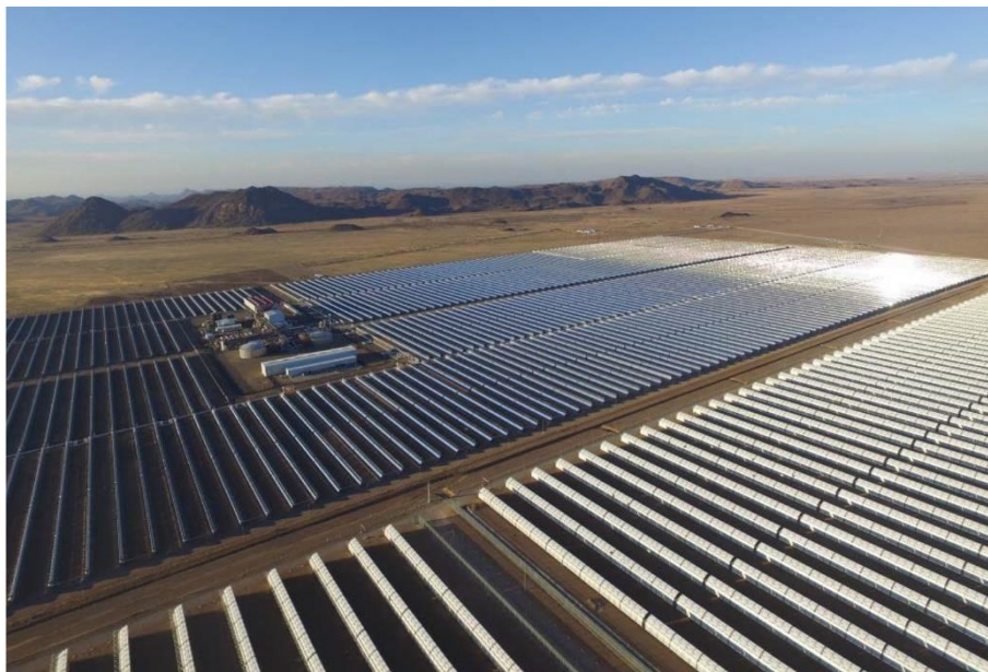
Figure 6.1. Partial shading of the Xina and Kaxu parabolic trough CSP plants, Pofadder, South Africa [106]
