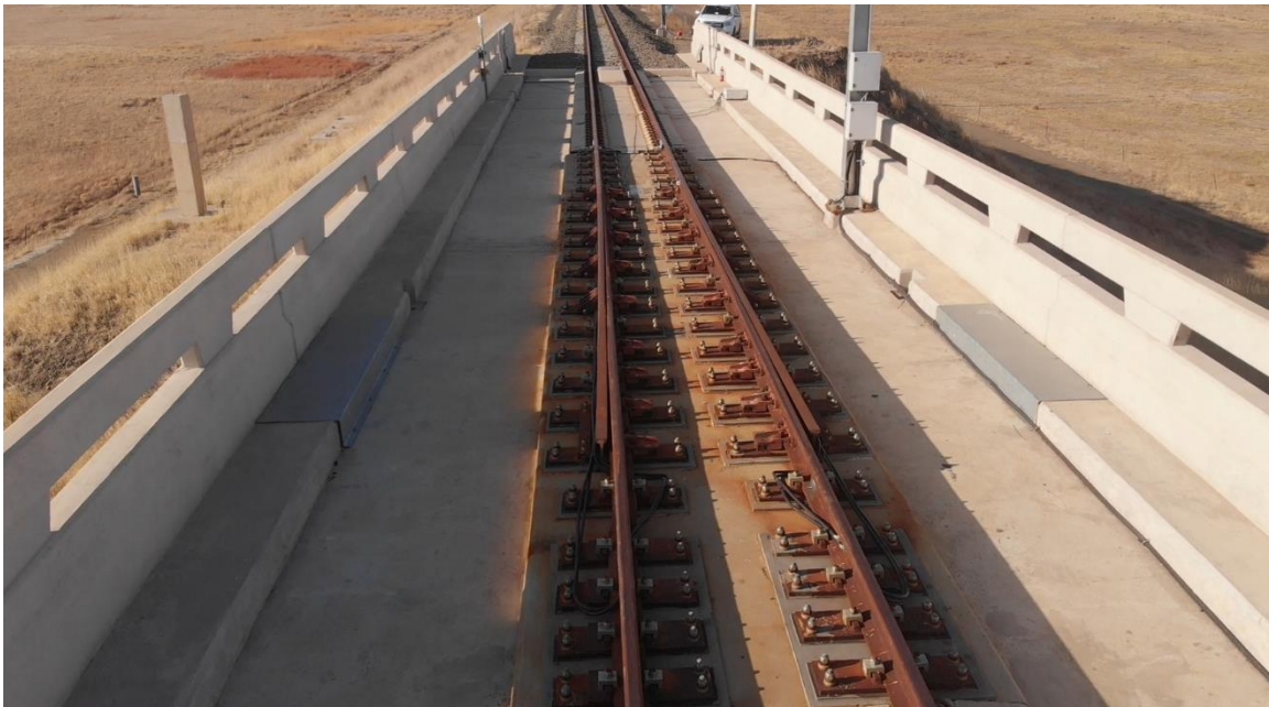
Figure 3.10: Rail Expansion Joint on Stage 3 Flat Track Slab
