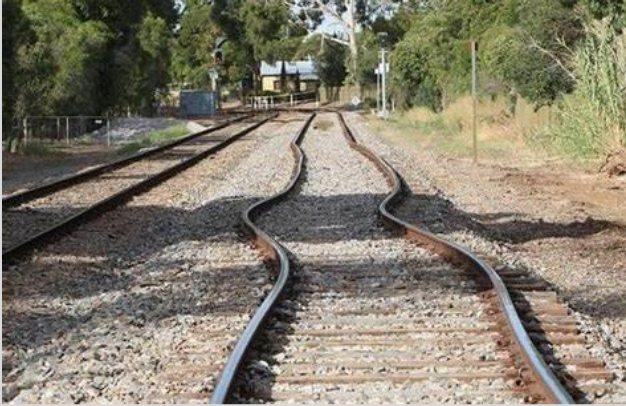
Figure 2.7: Rail kick out due to compressive forces
