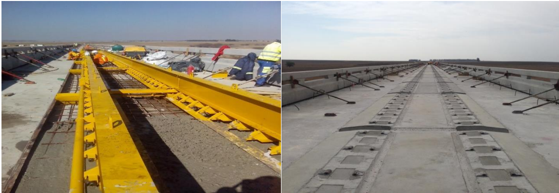
Figure 2.4: PY Track Slab construction (Photograph: Transnet Capital Projects)
