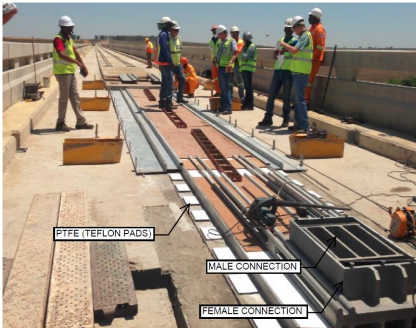
Figure 3.8: Construction of Stage 3 PY Track Slab
