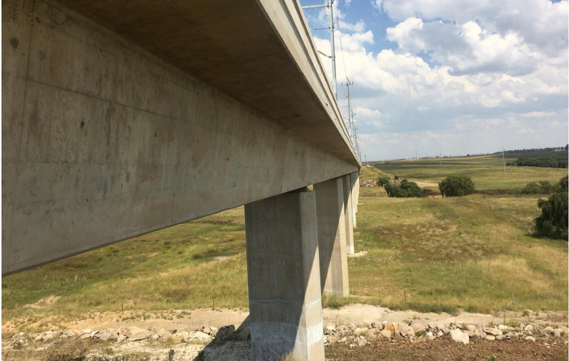
Figure 3.5: Majuba Rail Bridge Pot Bearings from Northern Abutment
