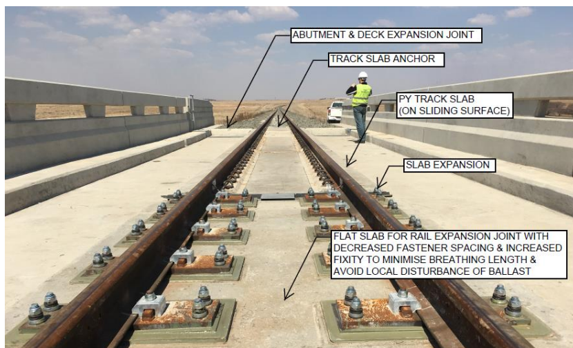
Figure 2.10: Rail Expansion Joint (Photograph: Transnet Capital Projects)
