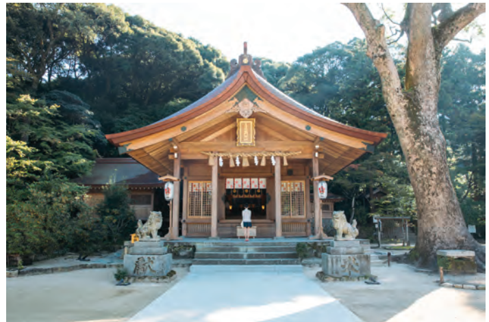
Figure S2.4 The Kamado Shrine in Dazaifu is surrounded by forest trees, in the tradition of shrine architecture. Visitors walk through a tunnel of trees to access the shrine. Starbucks Dazaifu sees the use of cedar as finding contextual synergy with this traditional context (dazaifutenmangu.org.jp, s.a.).
