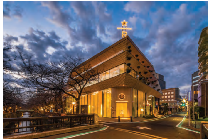
Figure S7.5 The terraced facade was designed in collaboration with Japanese architect, Kengo Kuma (Levy, 2019b)
