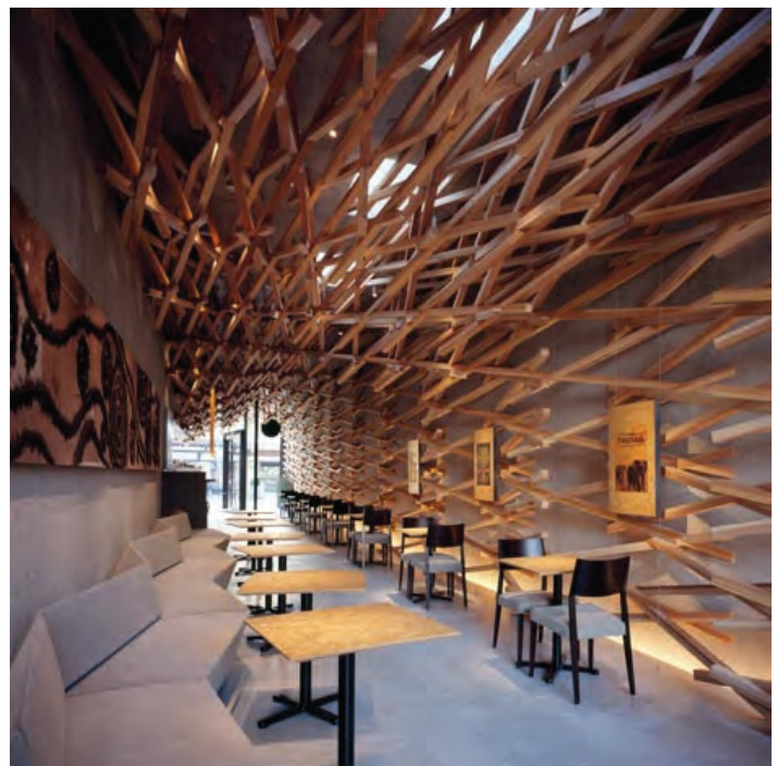
Figure S2.5 The store is constructed as a steel sheet, the interior is clad with an interwoven cedar stick structure that resembles a cedar forest (Frearson, 2012b)
