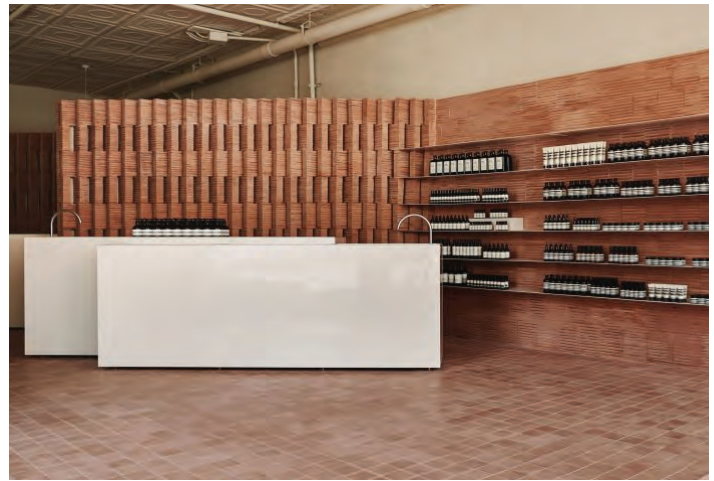
Figure A5.6 Existing pressed steel ceilings, masonry use and the diagonal layout reflect cues from the existing building and context (Cogley, 2019a)
