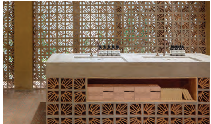
Figure A4.5 Cobogó brick used in multiple surfaces - floor inlays; counter and facade (taxonomyofdesign.com, s.a. [d])
