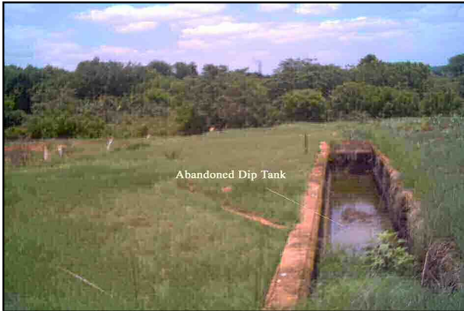
Figure 6.9 Disused Khubvi dip tank
