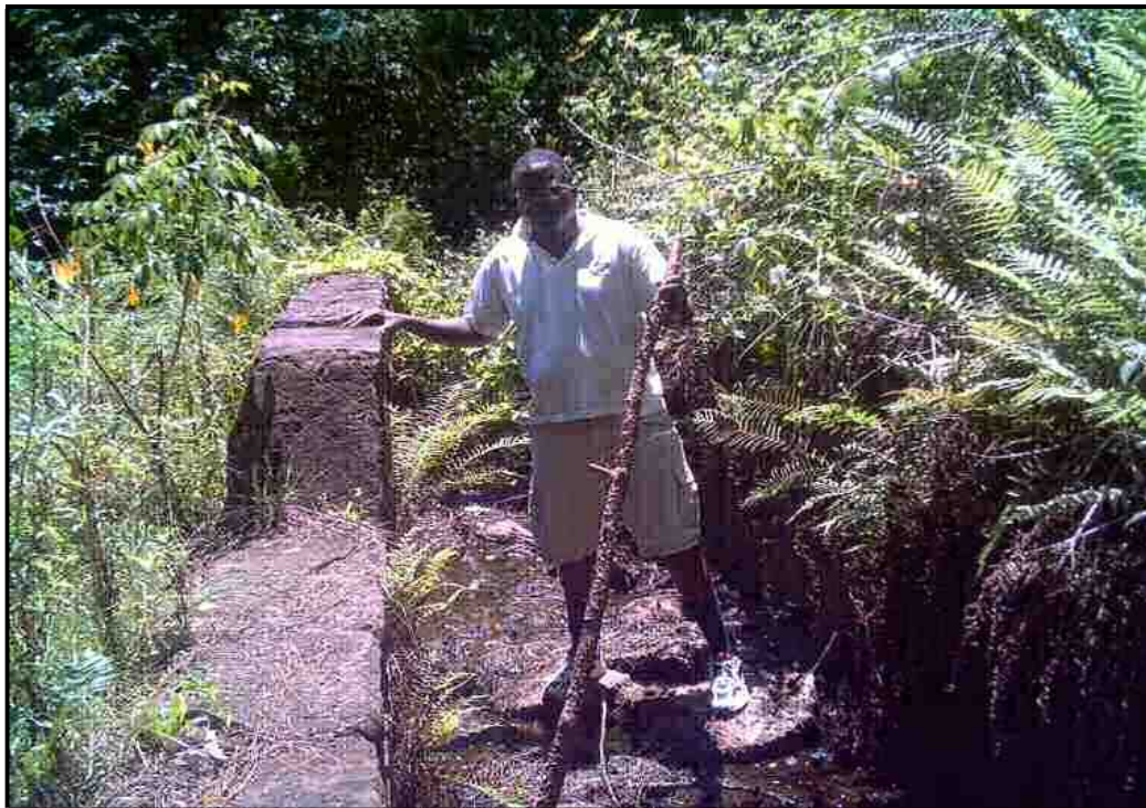
Figure 3.3 The ruins of the first dip tank established in Venda in 1915
