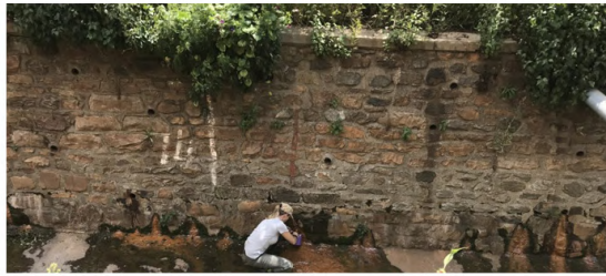
Due to the prevalence of sandstone that was generally excavated, many features have been built out of this material, most notably the sandstone river channel (built in the 1910s) which is also considered to be a protected heritage feature (Gumbi 2018).
