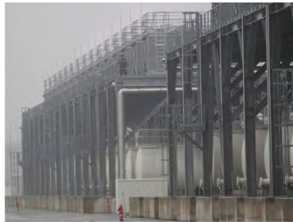
Figure 7.11 | Tanks containing coolant for servers at a Google data centre in Saint Ghislain, Belgium, which highlight the detrimental environmental effects of cloud computing. (Burrington 2015)
