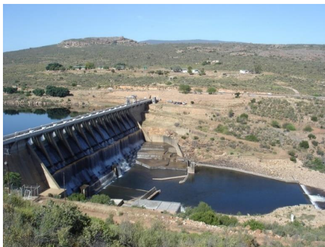
Figure 2-3: Clanwilliam dam (SANCOLD, 2021).
