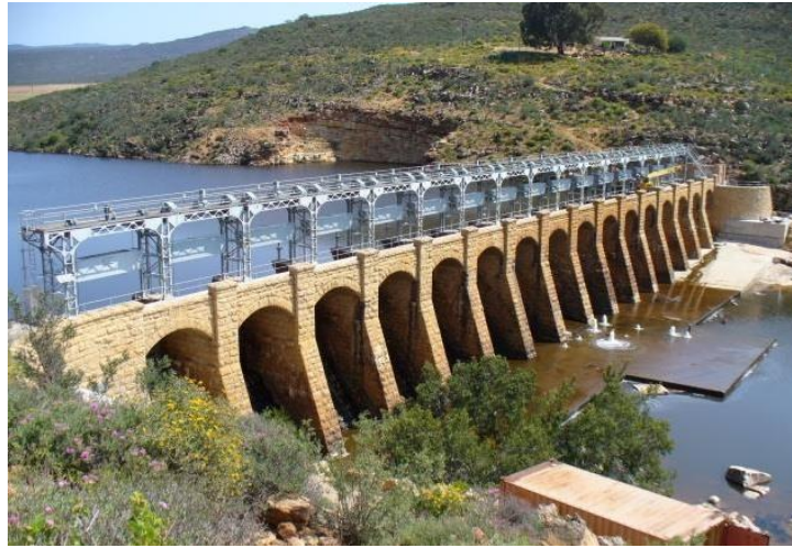
Figure 2-4: Bulshoek dam (SANCOLD, 2021).
