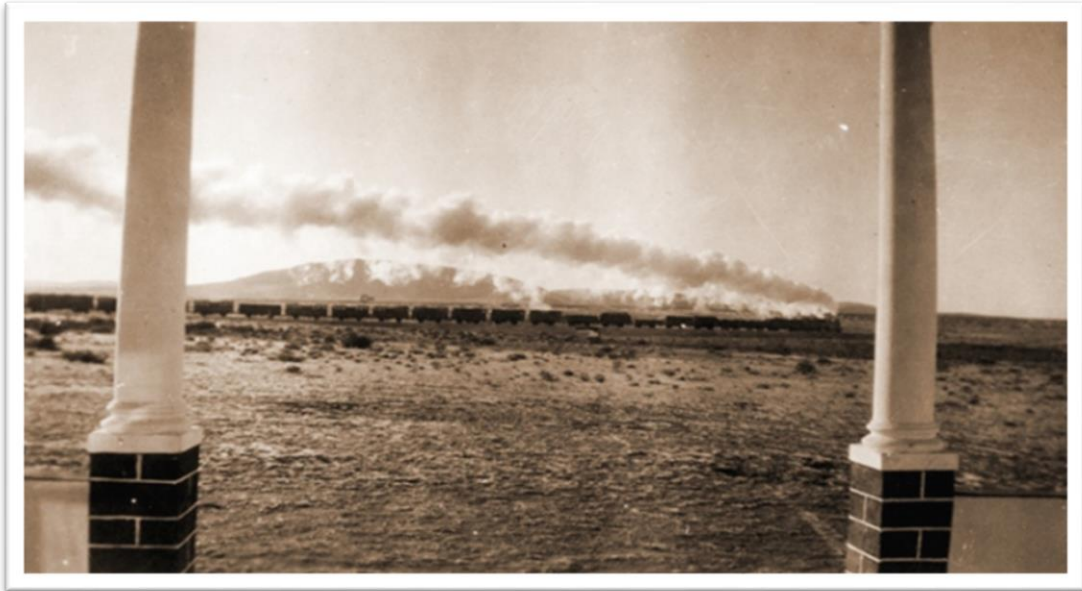
Figure 22: View of the railway track from our front stoep.
