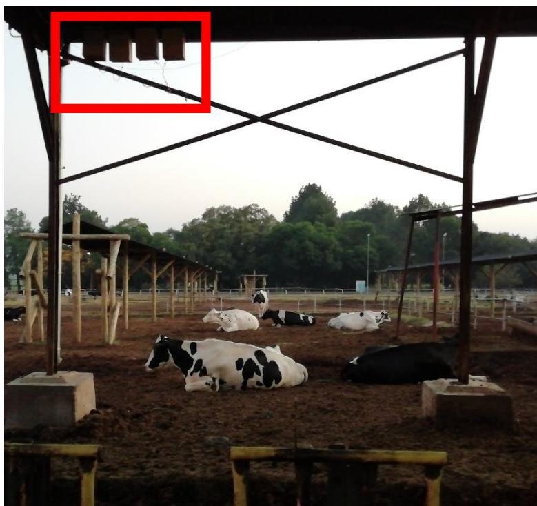
Figure 3.1 Four speakers in paddock area, two facing the feeding area and two facing the freestall section.
