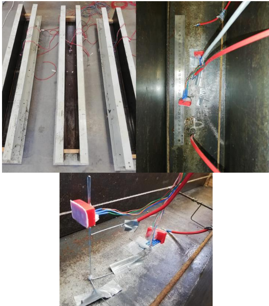
Figure 3.6: (Left) Thin pavement section moulds, (Right) relative humidity sensors and thermocouples spacing and (Centre) stand built to hold sensors
