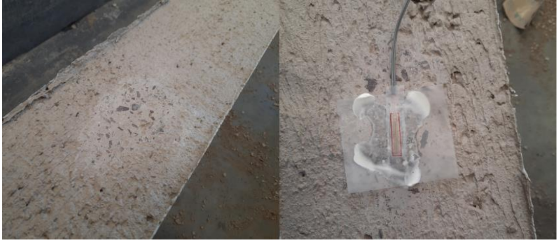
Figure 3.7: (Left) the preparation of the pavements surfaces and (Right) the HMB™ X60 adhesive bonding a strain gauge to the concrete
