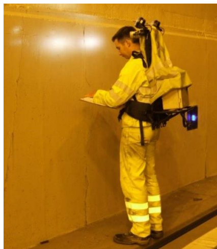
Figure 2.4: Visual assessment with additional lighting (CETU, 2015)
