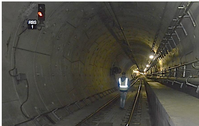
Figure 3.26: Capturing of point cloud data in TBM tunnel section
