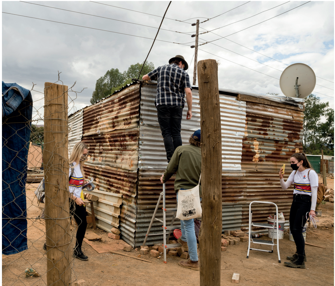
Figure 2.41: Installation of sensors and structured observations in Melusi with BArch Honours students (Eyescape 2021).
