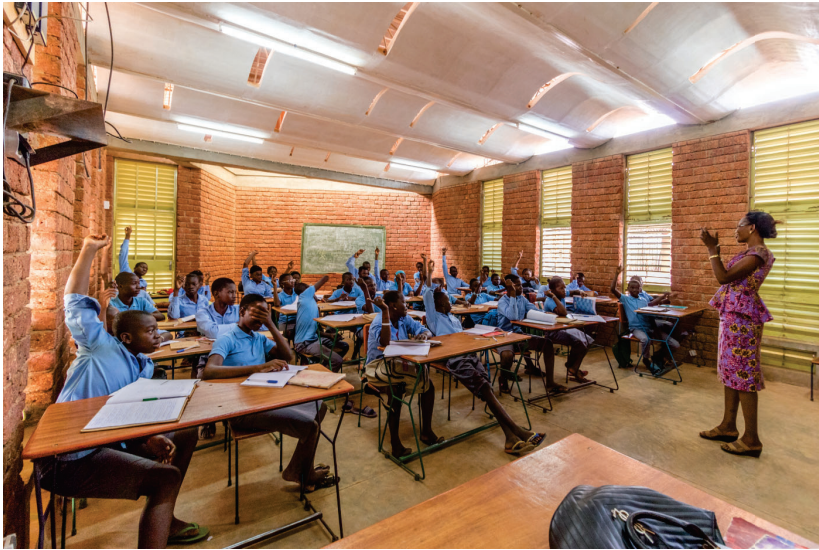
Fig 93: Photograph showing perforated plaster vaults (Kere Architecture 2019)
