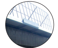
Steel Frames with Bracing
