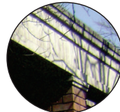
Concrete Up-stand Beams
