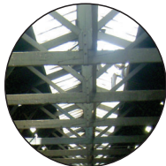
Steel Roof Trusses
