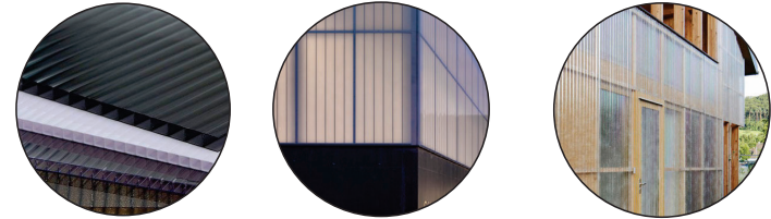
1. Polycarbonate sheets of various transparencies Steel sections will be used to create the various frames that will be arranged to create various patterns.
