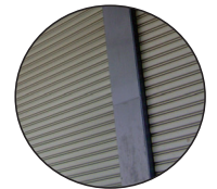
Steel Sheetting facade infill steel frame
