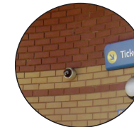
Contrasting Face-brick Walls
