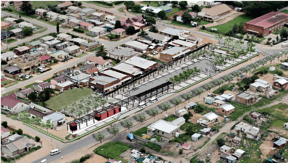
Bird's Eye View showing how the development sit in the context and how it relates to its surroundings. (New
