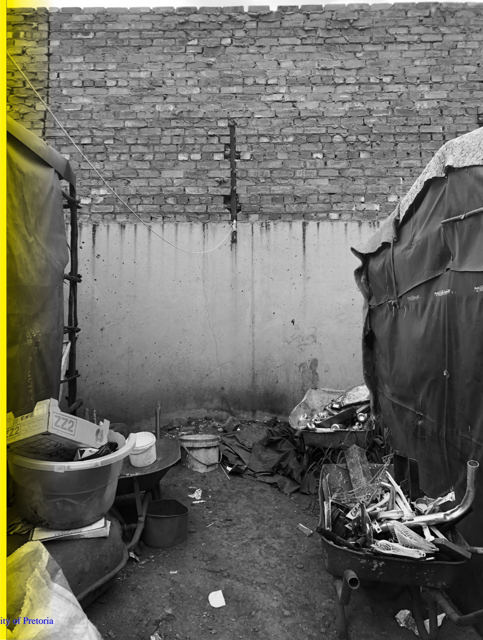
Figure 1.0.1: (right) Boundary wall in Cemetery View, Moreleta Park (Author 2020).
