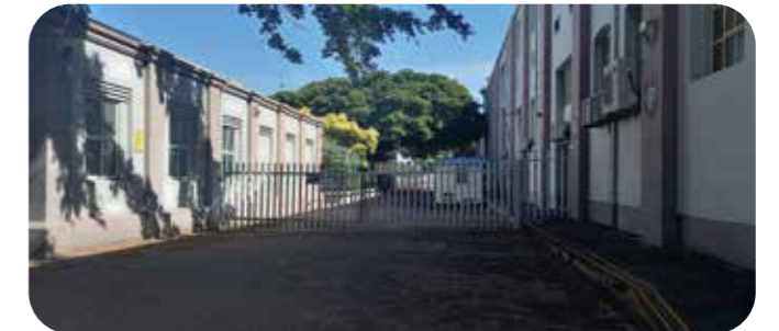
Figure 3.30 'Fenced off site' (Author, 2021)
