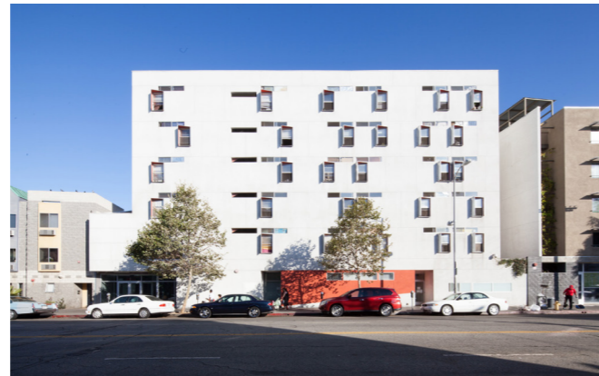
14.3. Photograph of southern (street) elevation (Maltzan 2020).
