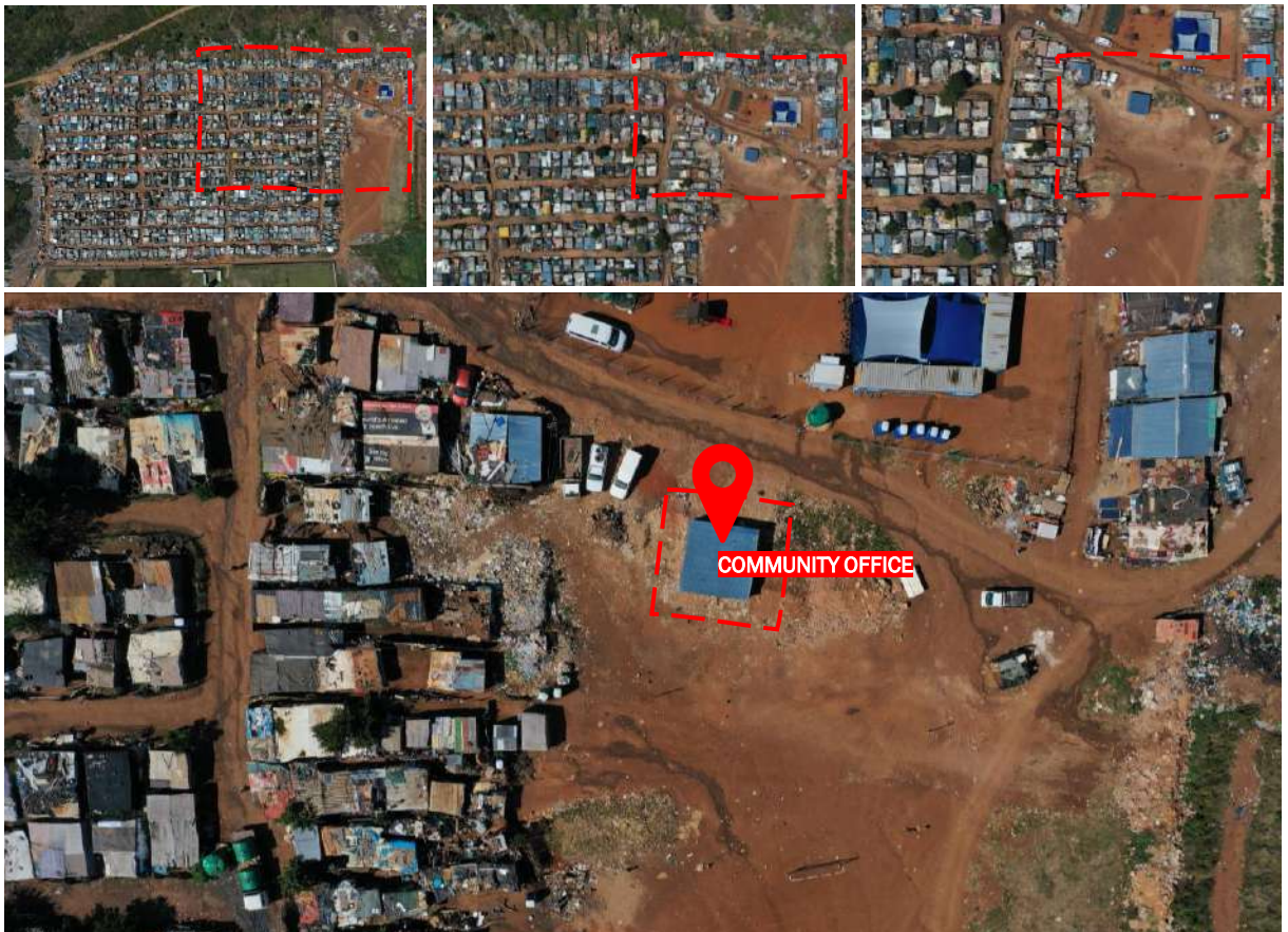
Figure 12: The community office was located on the edge of the informal settlement and is known among the community as a safe space for mediation, knowledge transferal and expression (Moreleta Park Integration Project, 2021).
