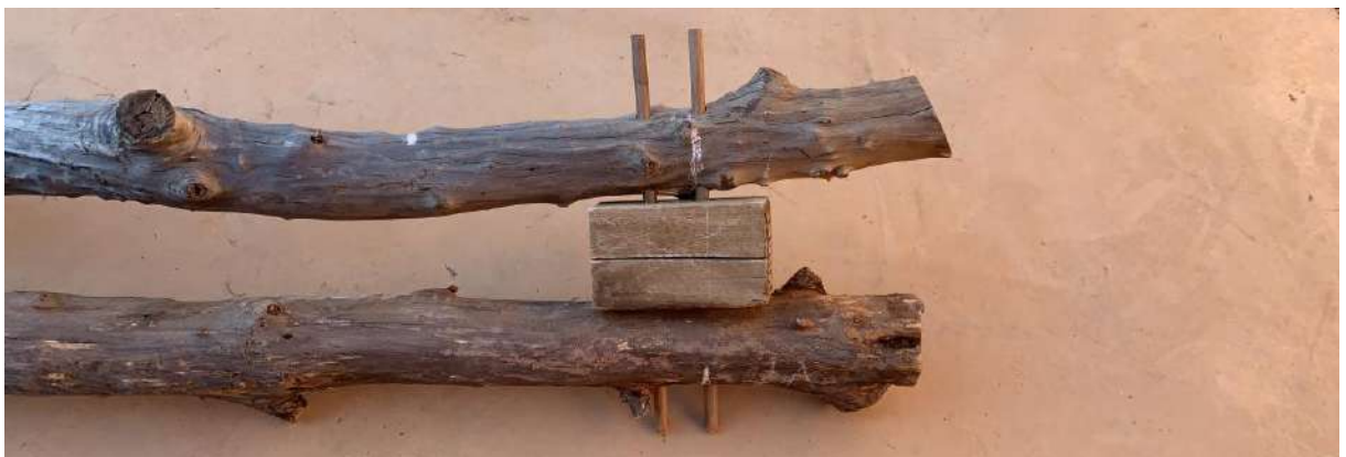
Figure 51: Fixing method that showcases a bridge between 'bottom-up' and 'top-down' approaches by using materials found on site and applying expert knowledge (the 100mm spacer) to ensure structural integrity (The Moreleta Park Integration Project, 2021).
