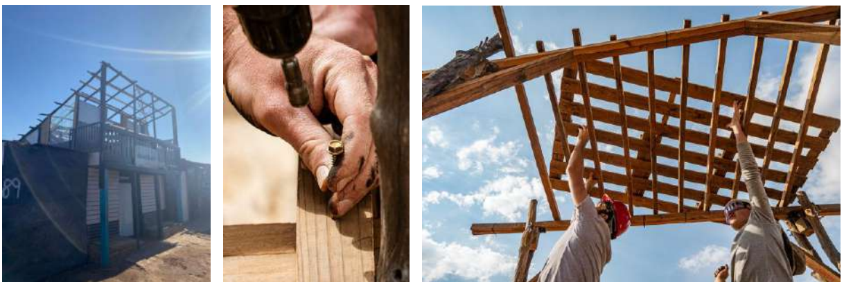
Figure 53: The prototype's intention on site was to serve as a precedent of structural interventions that can be built with materials that can be sourced from the settlement. The photograph in the left is a structure that was built after the prototype and used the contrition methods to build a double storey (The Moreleta Park Integration Project, 2021).
