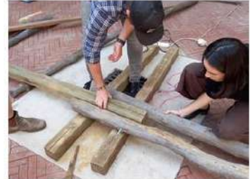
A prototype built by the Moreleta Park Integration Project to develop a method of constructing with uneven elements (MPIP, 2021).
