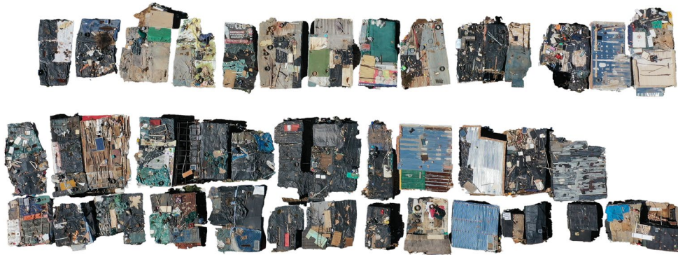
Figure 1.4 - Informal housing roofing photo, (MPIP, 2021)
