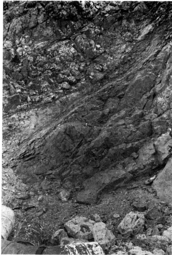
Plate XIII. Thrust shear plane on the western sidewall of the -1400' slot. Note the intense brecciation in the hanging-wall which lowers the stability of the slope.
