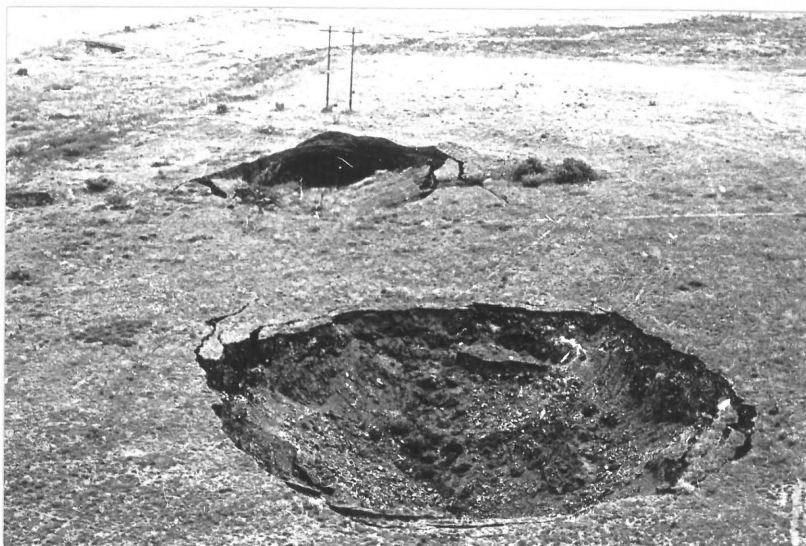
foto 7 SINKGATE IN DIE WONDERFONTEINSPRUIT AS GEVOLG VAN ONTWATERING.
