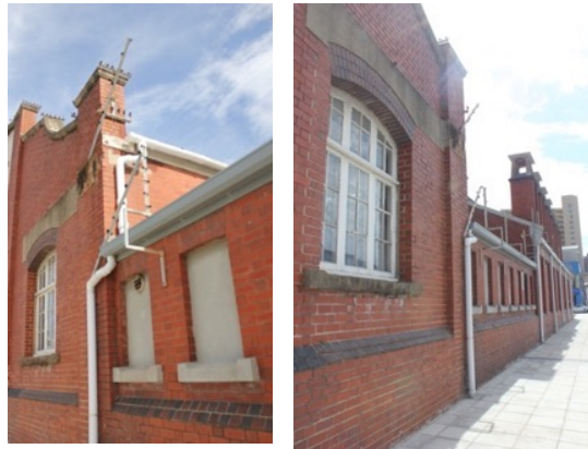
Figure 101-102: Brick plinth on southern façade (Author 2021)
