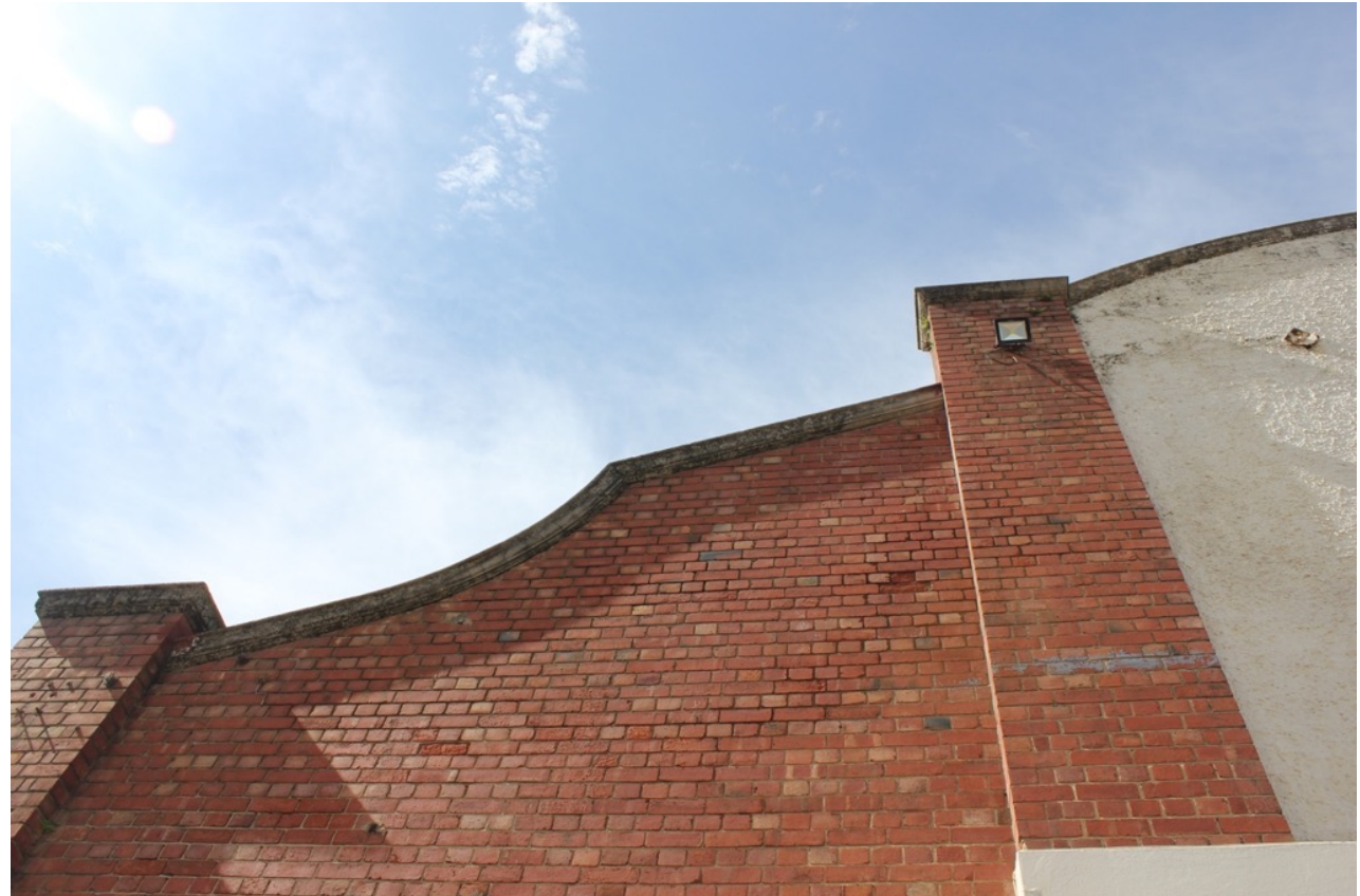
Figure 60: Gabled façade and brick detailing, Rivertown Beerhall (Author 2021)
