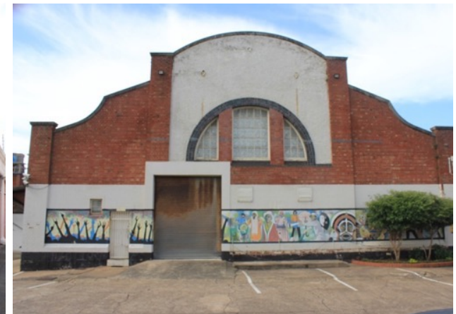
Figure 108: North Facade (Author 2021)
