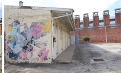
Figure 87: Out building (Author 2021)
