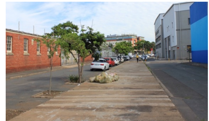
Figure 113: Covered canal (Author 2021)
