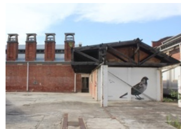
Figure 86: Courtyard & Plant Room (Author 2021)
