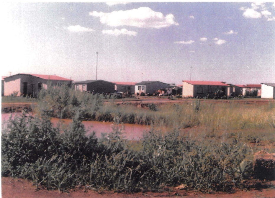
Plate 8: Poor drainage on portion of township.
