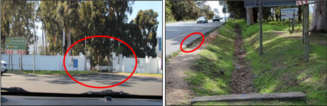
Figure 8: Examples of observed risk factors at intersection of R45 and R310 (2019)
