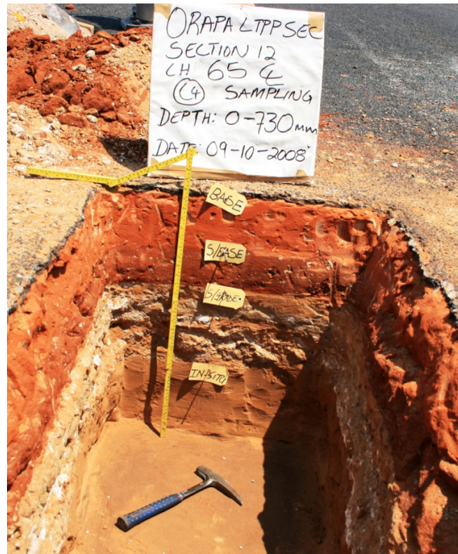
Figure 1: Profile at CH. 65 CL on Section 12 (Photo: Mr S Pilane)
