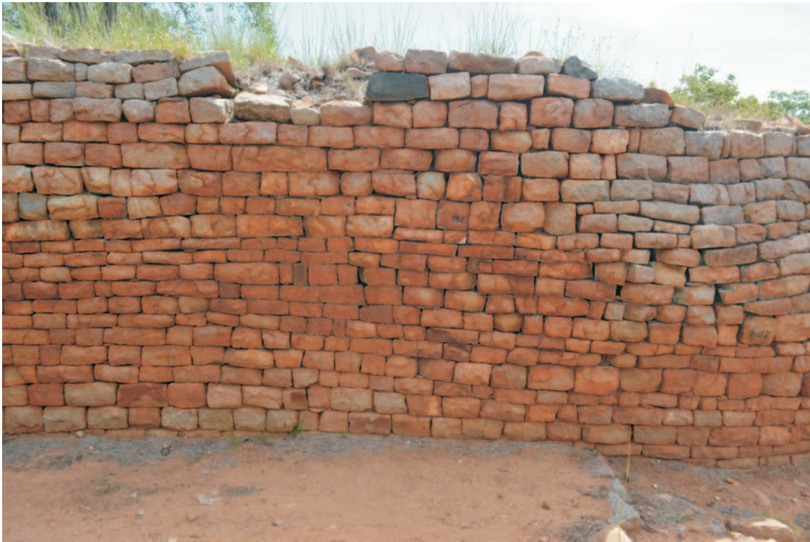
FIG. 9. Bonded and interlocking walling at Khami site.
