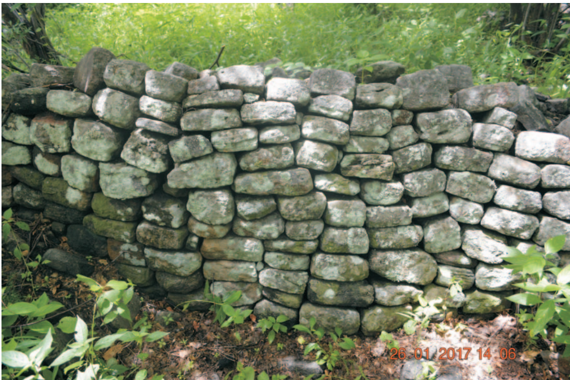
FIG. 8. Shangano wall straight joints.
