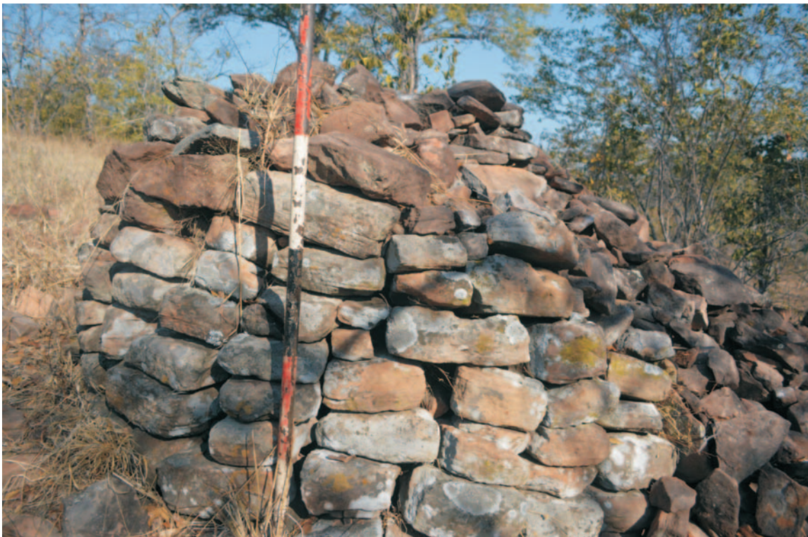
FIG. 10. Vertical joints at Halfway House site.
