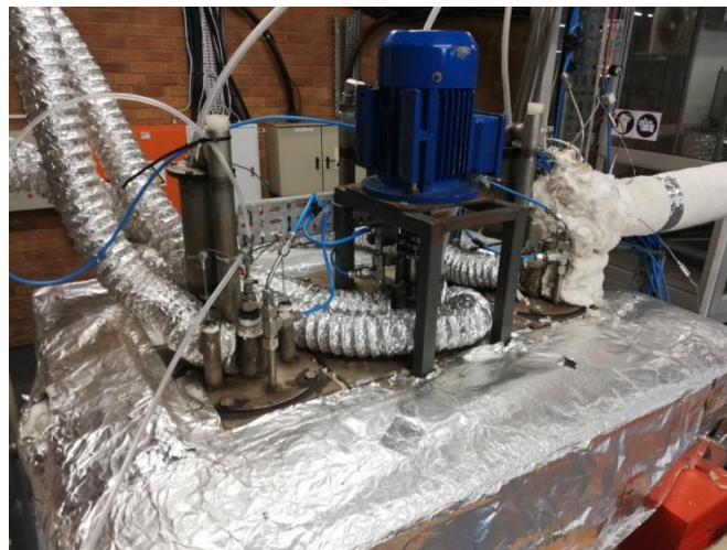
Figure 56: Photograph showing an overview of the reactor's lid
