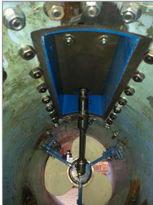
Figure 3-22: Modified Kaplan prototype turbine (prototype 2) – interior view
