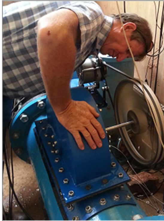
Figure 4-17: IPW2 retrofitted on the installed baseplate
