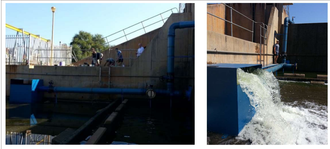
Figure 2-15: Zeekoegat installation – type 2, island syphon
