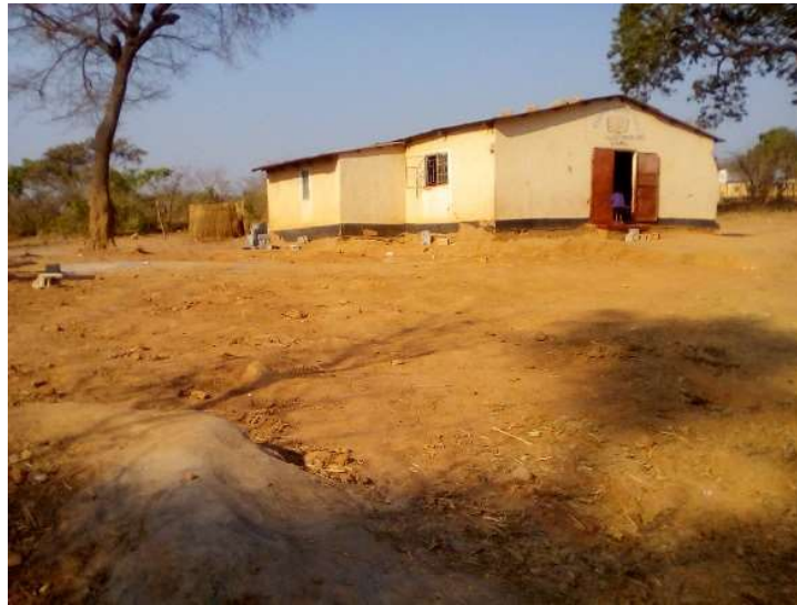
Photograph 5.13: Chipego school building
