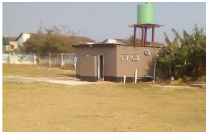
Photograph 5.2.2: School water tower and ablution block
