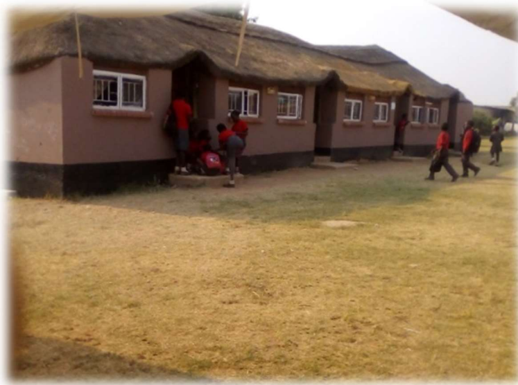
Photograph 5.2: Chitukuko school block
