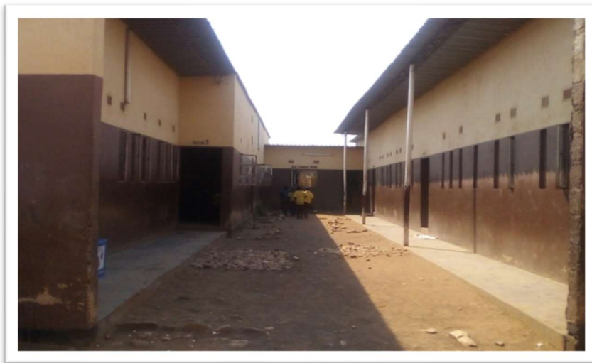
Photograph 5.9: Chifundo school blocks (front) connected by head teacher’s office (back)
