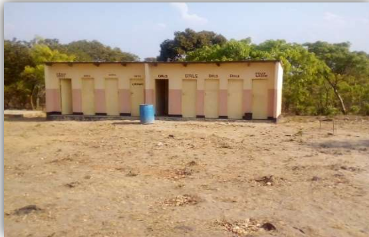
Photograph 5.3: School ablution block
