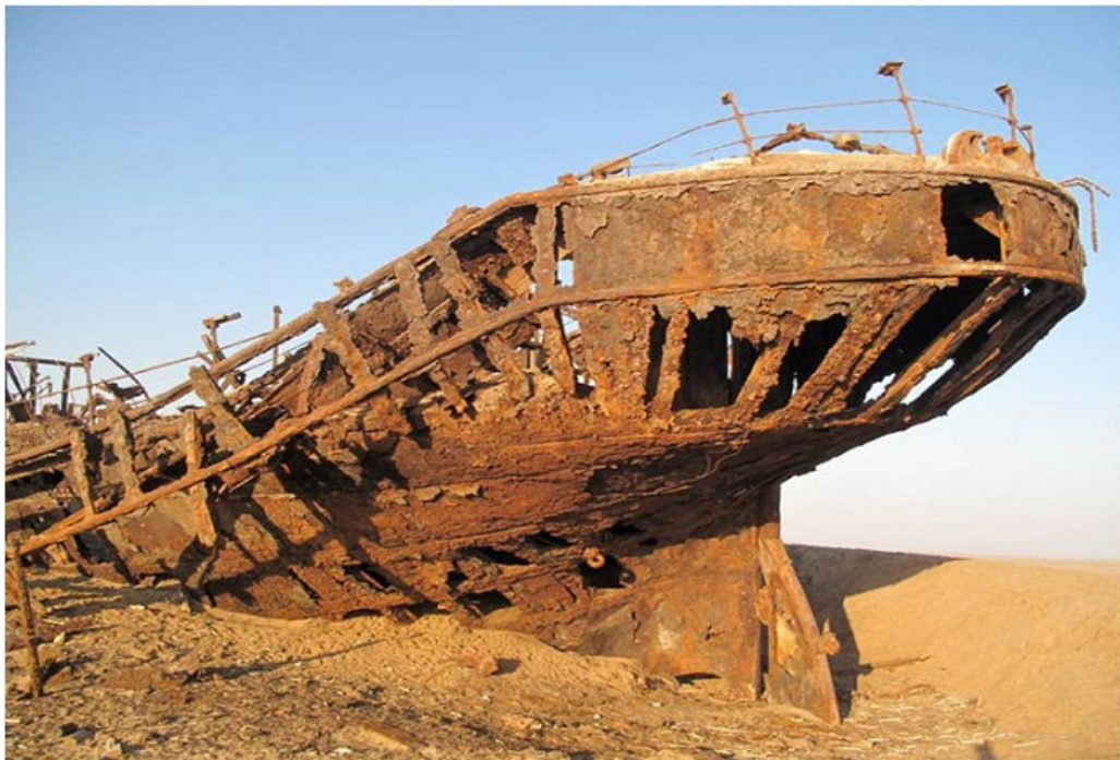
Figure 6.5. Collapsed Guard rail and severe corrosion of the stern side, including the rudder of Eduard Bohlen (Source: Harris et al. 2012).
