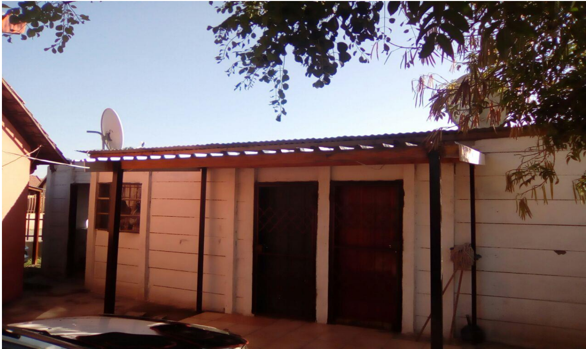
Photograph 11: Two backrooms made of precast in Million Dollar, Rustenburg. 10 November 2017.
