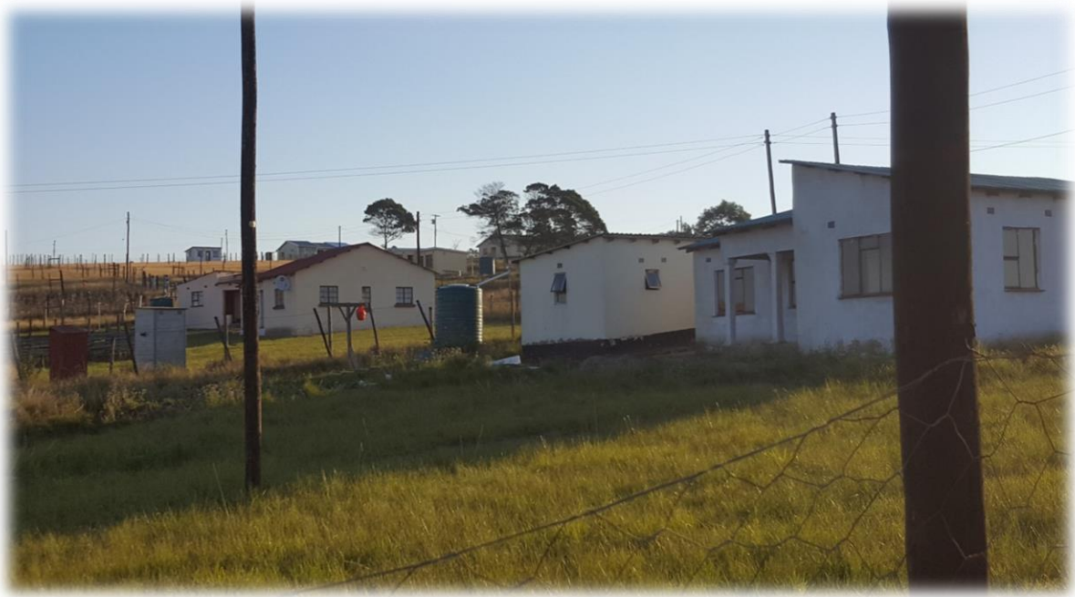
Photograph 17: Houses of mineworkers in Ngobozane, Lusikisiki
