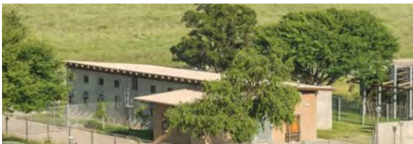
The new Wildlife Clinic, an expansion of the Onderstepoort Veterinary Academic Hospital at the Faculty of Veterinary Science
