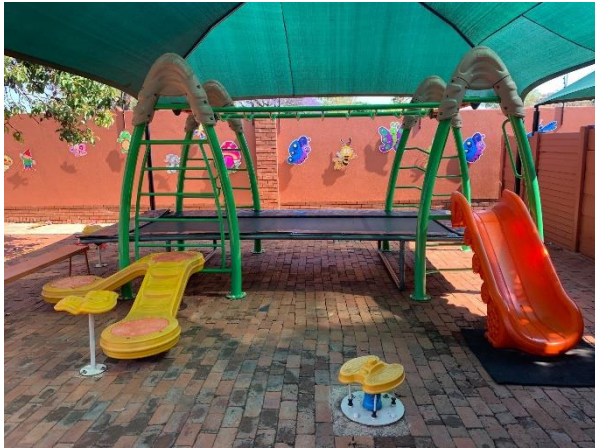
Photograph 4.9: A steel frame at ELC3
