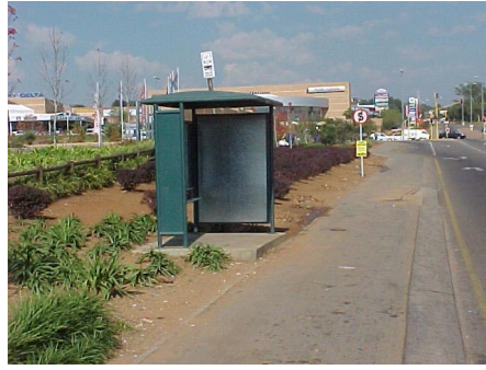
Figure 2: Typical Public Transport Shelter in Pretoria
