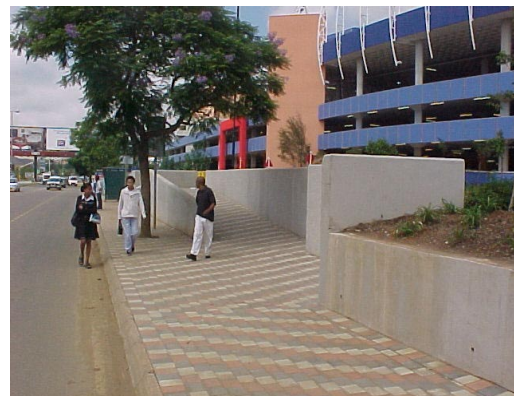
Figure 8: Ramps and Sidewalk on Lois Road
