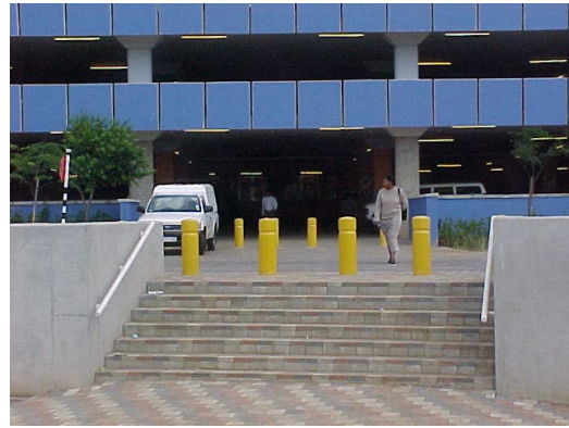
Figure 10: Staircase on Lois Road
