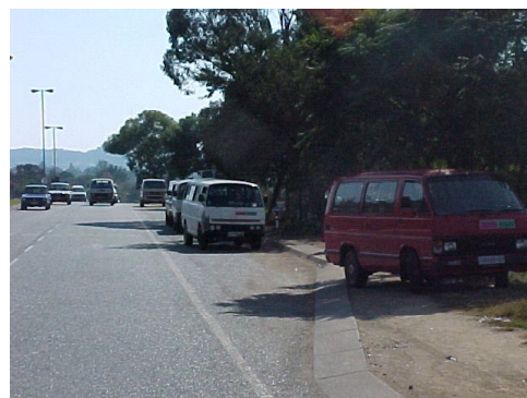
Figure 4: Unpaved Sidewalk on Atterbury Rd
