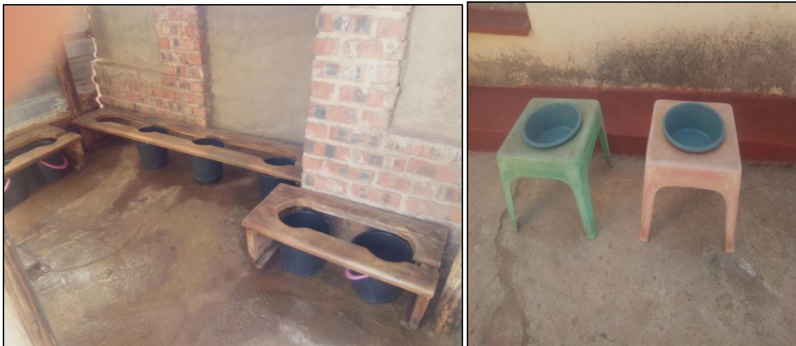
Photograph 4.9: Children's toilets and hand washing basins at Centre B (rural area)
