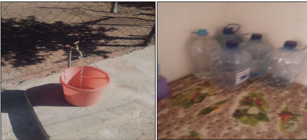
Photograph 4.10: One tap of running water and containers at Centre B (rural area)
